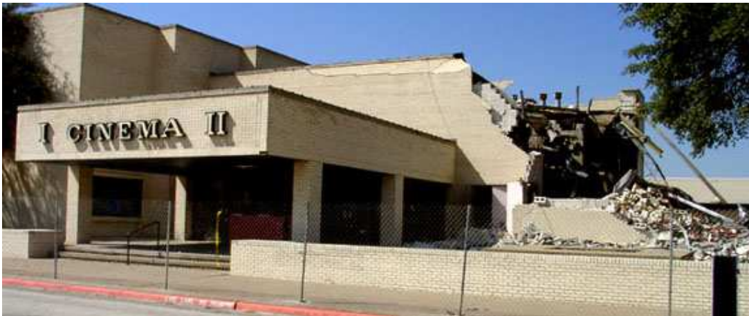
Figure 30 - Demolition of Cinema II
