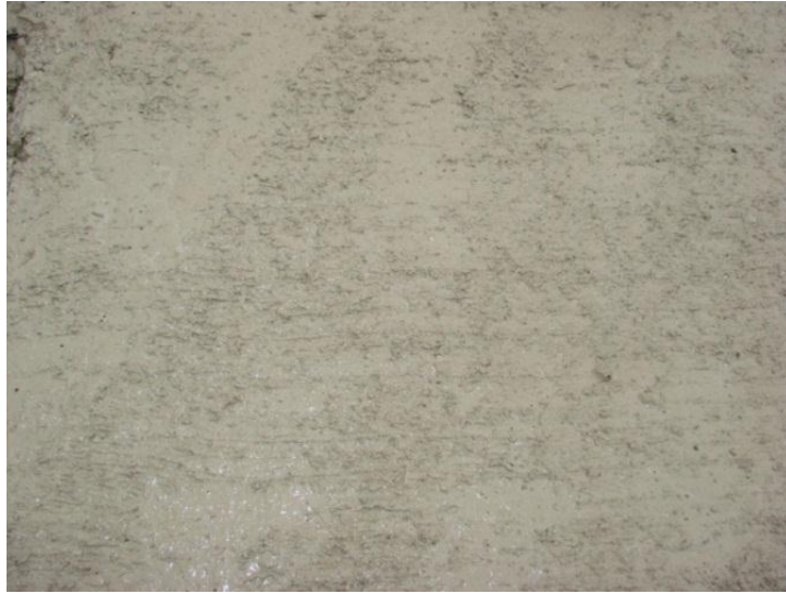
Figure 3-15 Surface finish on precast panel
