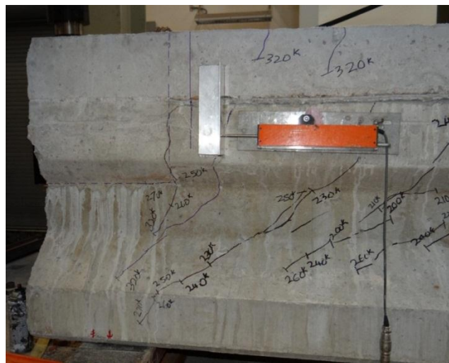
Figure 5-63 Shear cracks and interface cracks near the southeast support
