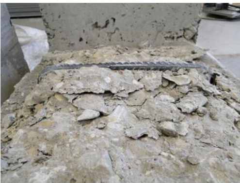
Precast failure plane
