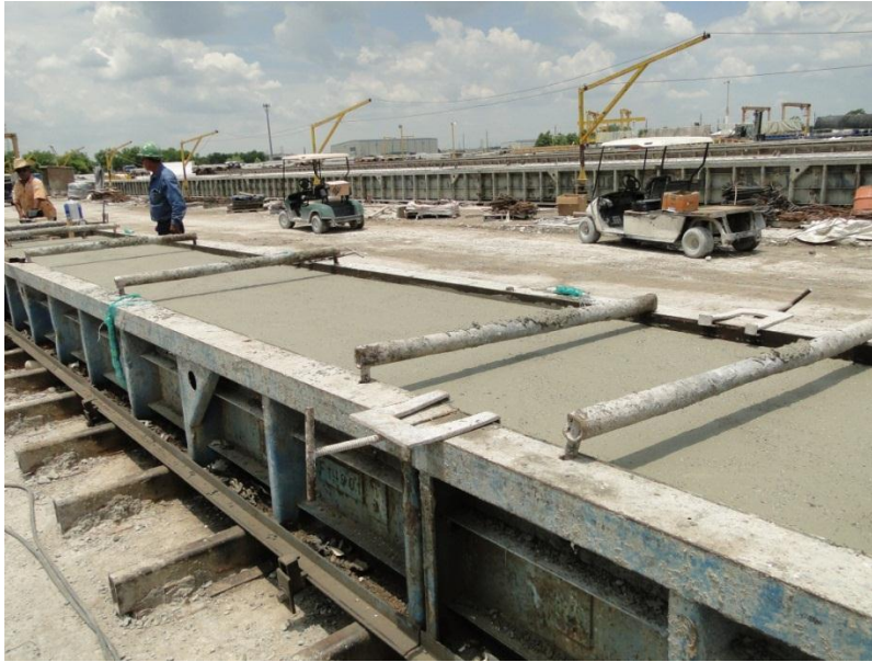
Figure 4-96 Finished CIP slab
