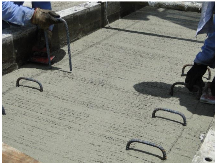
Figure 4-54 Placing of horizontal shear reinforcement
