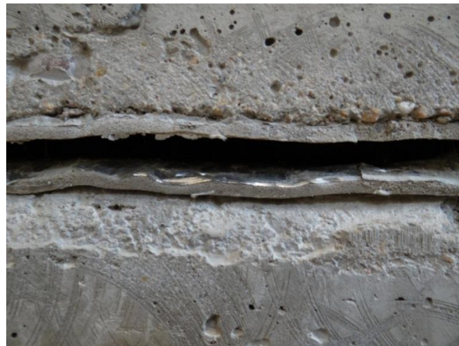
Figure 5-46 Separation between CIP slab and precast beam
