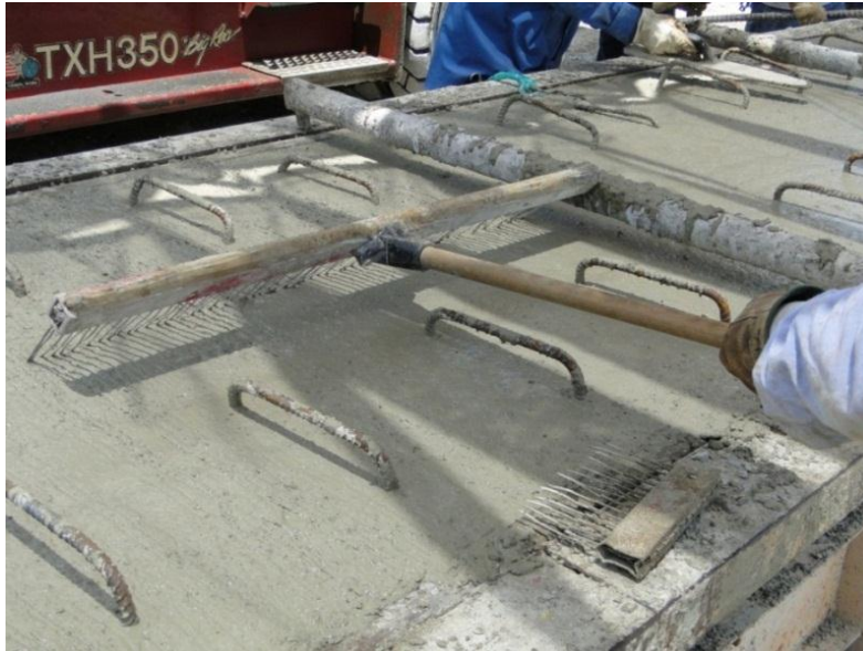
Figure 4-47 Rake finish on box beams
