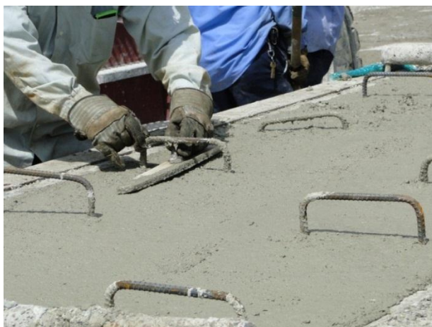
Figure 4-76 Wood float finish
