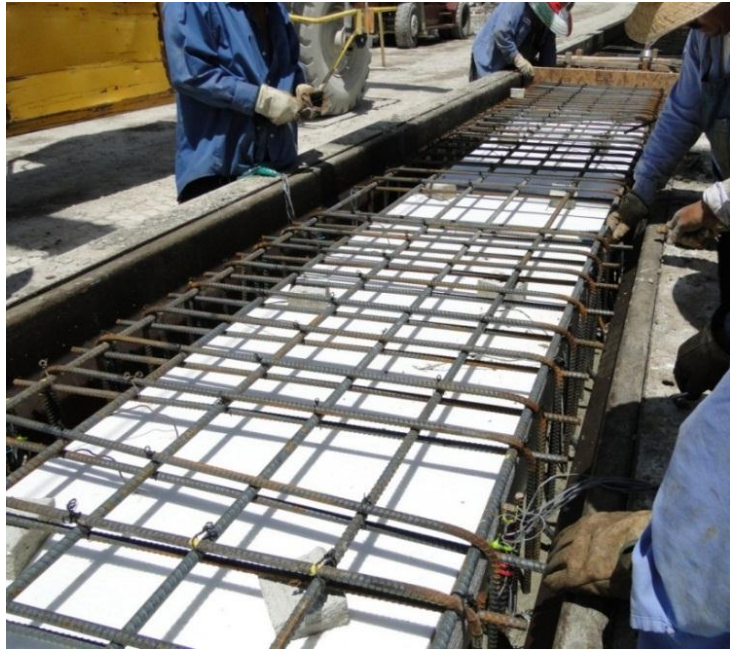
Figure 4-45 Top reinforcement for box beam without horizontal shear reinforcement
