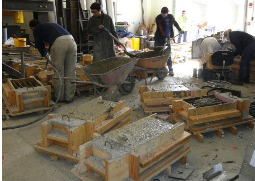
Figure 4-29 Casting of CIP part of specimens
