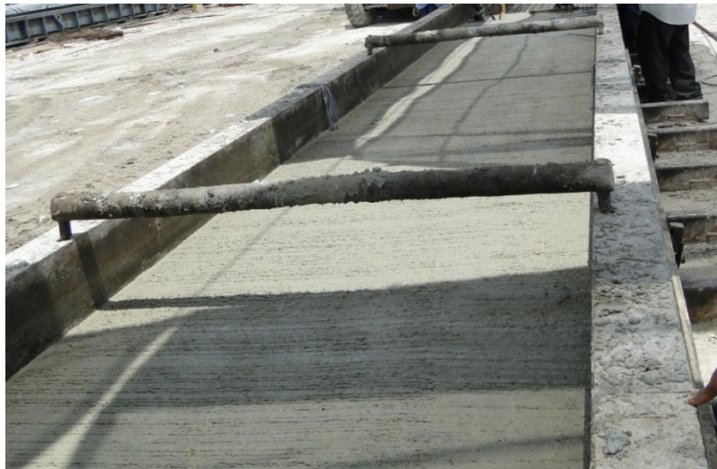
Figure 4-56 Finished slab beam without horizontal shear reinforcement
