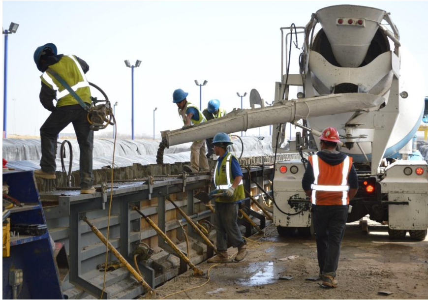
Figure 3-17 Casting of I-girders
