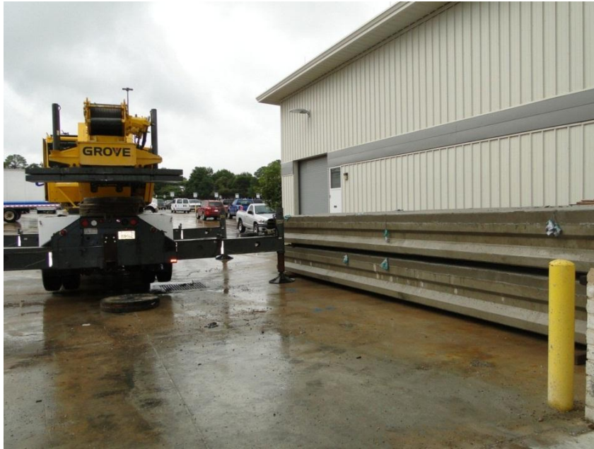
Figure 4-71 Storing of the beams outside the lab
