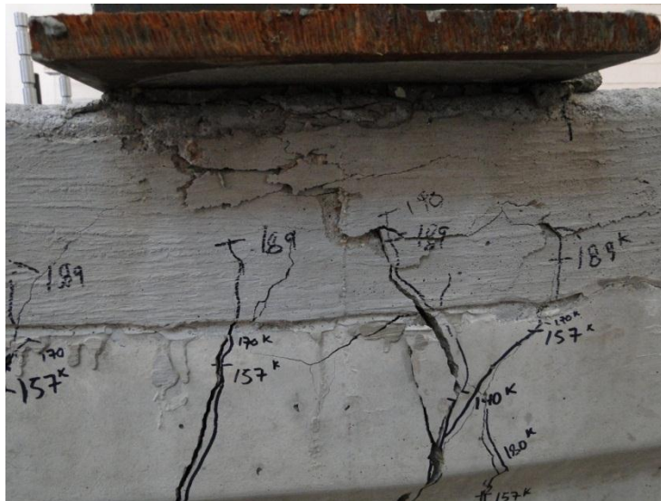
Figure 5-25 Concrete crushing at failure
