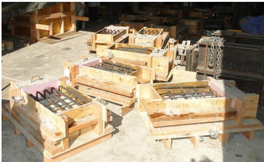
Figure 4-28 CIP caging and formwork
