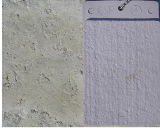
Figure 3-10 SCC concrete surface compared to CSP 4
