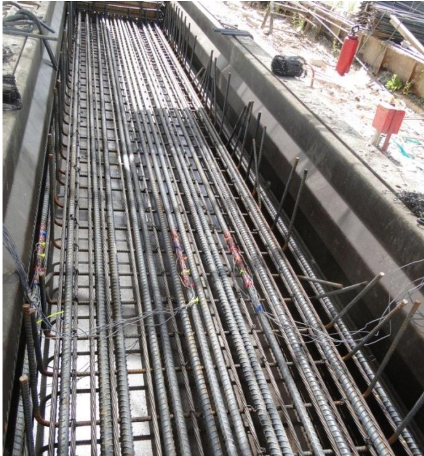
Figure 4-41 Reinforcement layout
