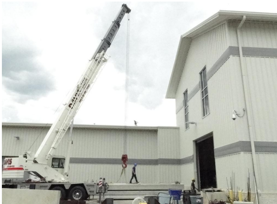
Figure 4-97 Storing of the beams outside the lab
