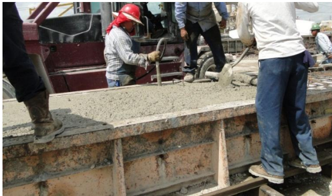
Figure 4-75 Casting of the top part of the box beam
