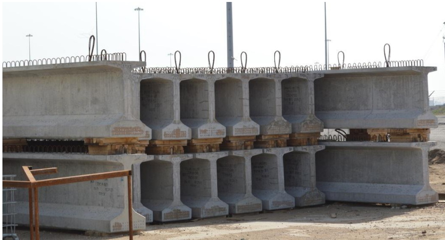
Figure 3-16 I-girder fabricated by Atesvi US
