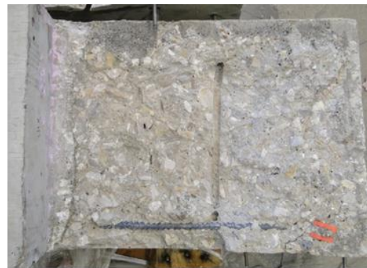
CIP slab failure plane
