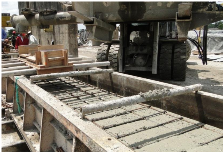
Figure 4-82 SCC Slab beam casting
