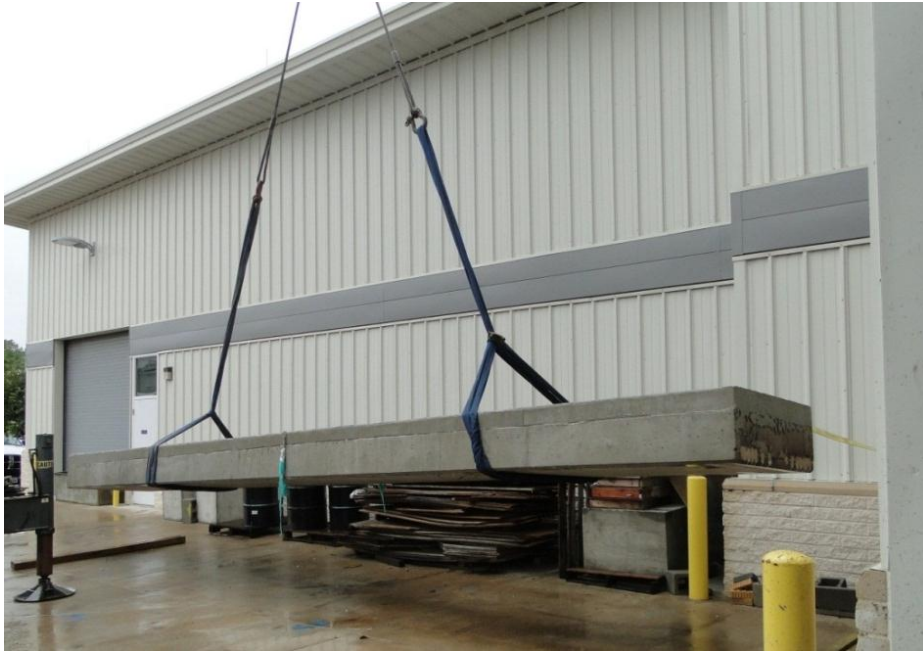
Figure 4-69 Unloading of slab beams
