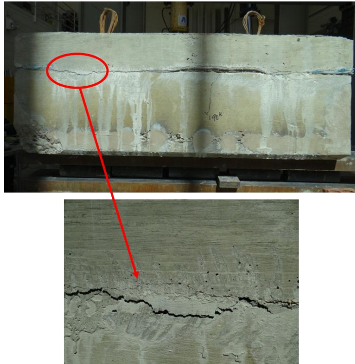
Figure 5-44 Cracking at the interface (photo taken at the beam end)
