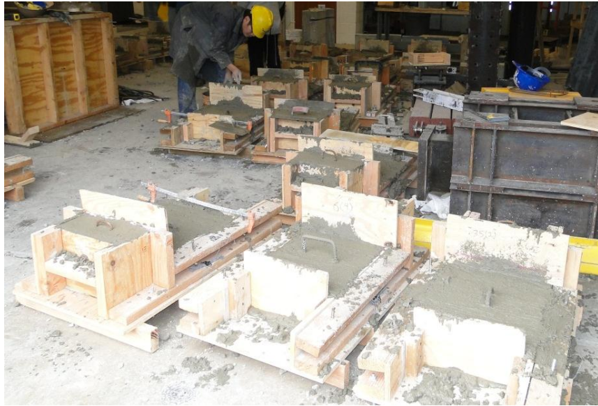
Figure 4-27 Completed precast section casting
