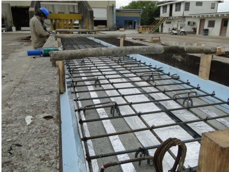
Figure 4-94 Foam tape on the box beam
