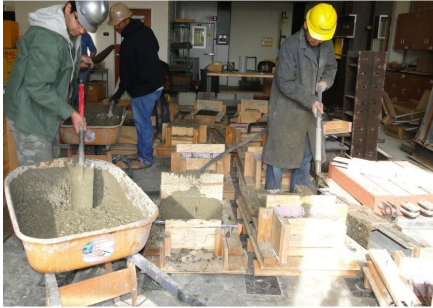
Figure 4-25 Casting of the precast section
