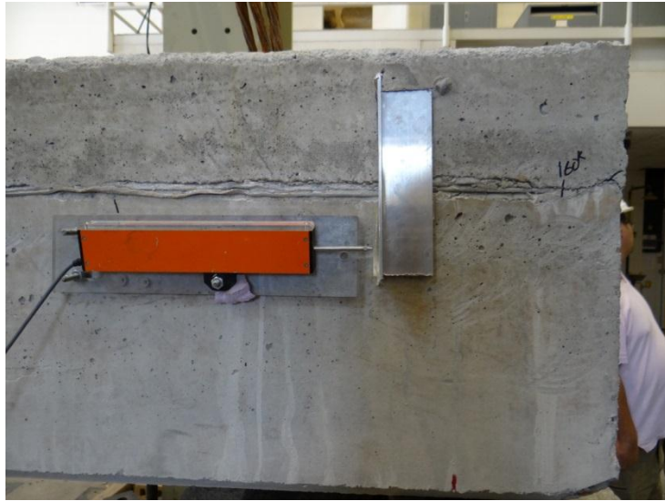
Figure 5-37 Visible interface cracks East-edge of beam
