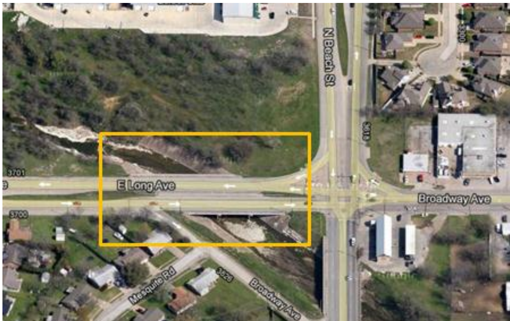
Figure 3-3 Location of Long Ave. Bridge
