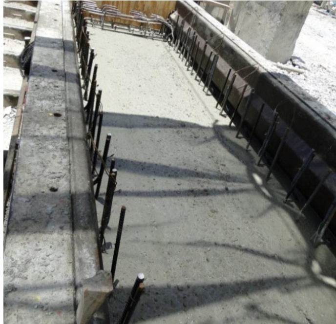
Figure 4-42 Concrete poured to 5-in.
