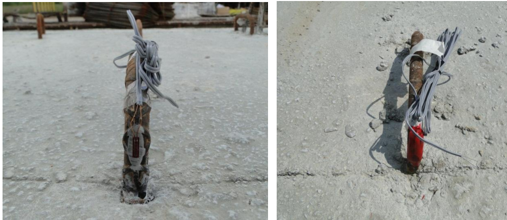
Figure 4-90 Strain gauges installation on horizontal shear reinforcements
