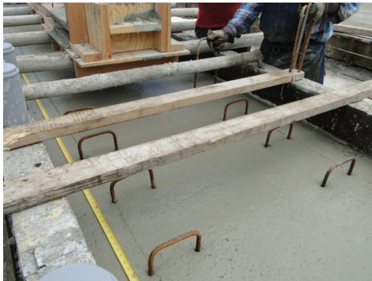
Figure 4-84 Placing of horizontal shear reinforcement
