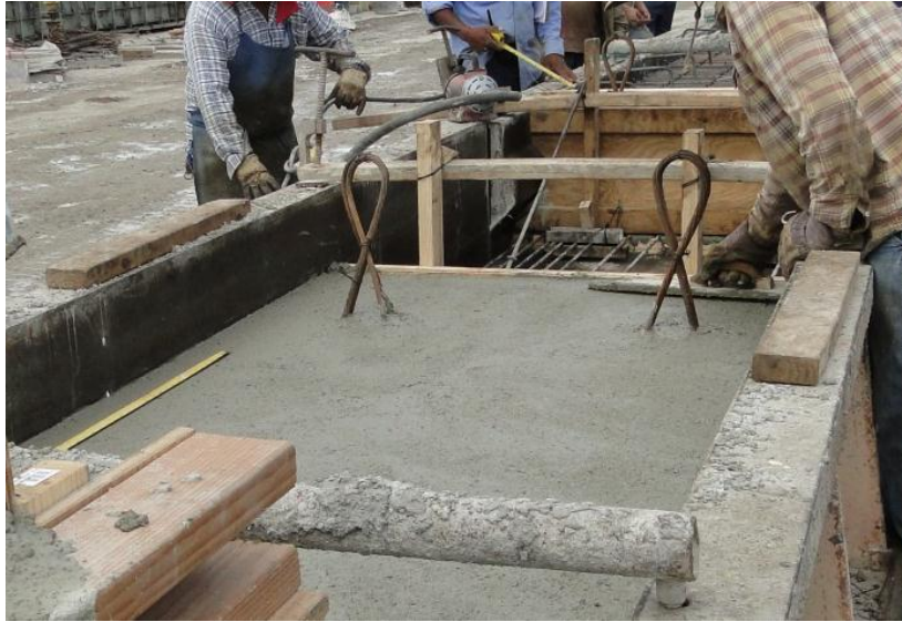
Figure 4-83 Wood float finish
