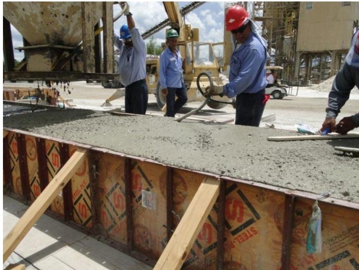
Figure 4-66 Vibrating and wood float finishing
