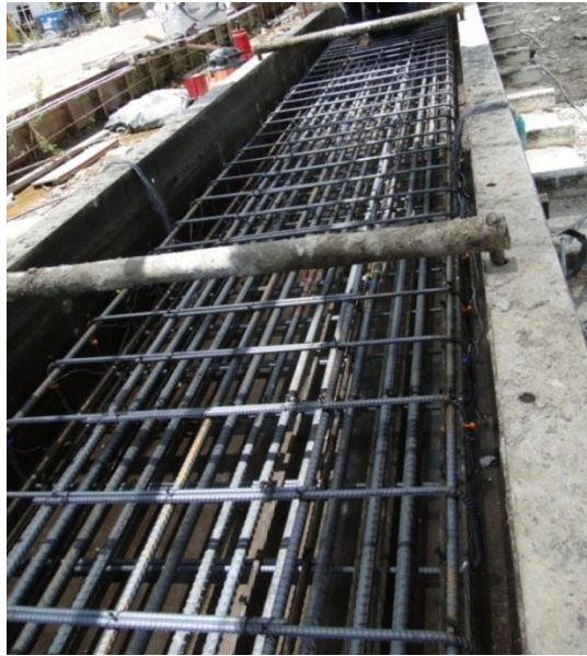
Figure 4-81 Finished slab beam reinforcement
