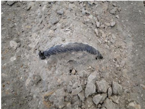
Precast failure plane
