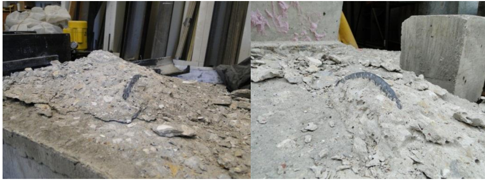
Figure 5-2 Task 4 (a) 3.5"-180° and (b) 3.5"L-180° failure plane showing bar pullout from the CIP slab
