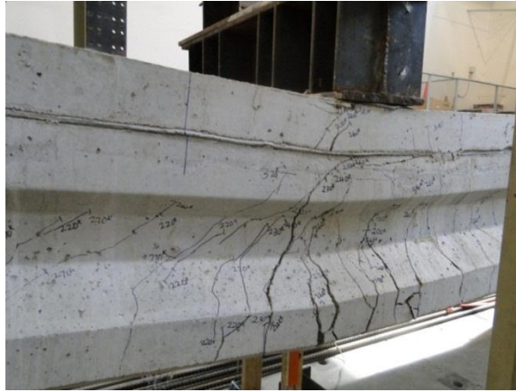
Figure 5-66 Failure of specimen (side view)
