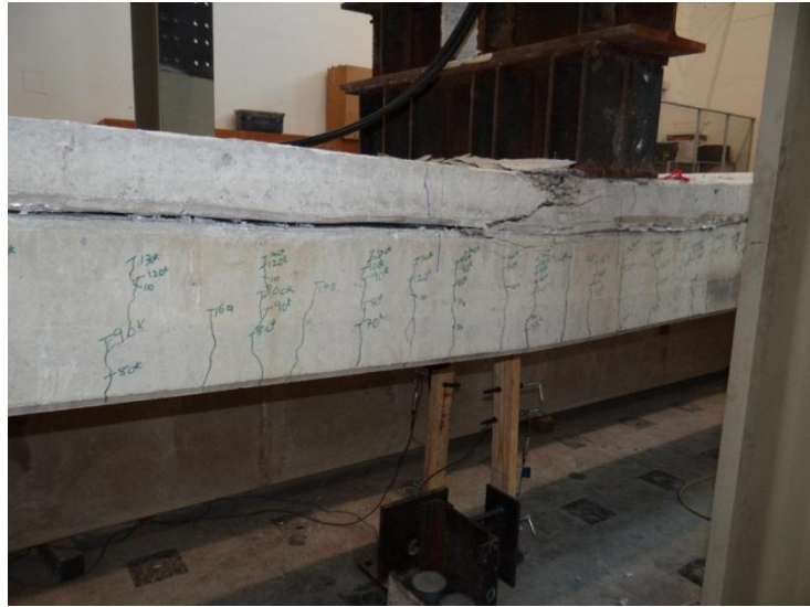
Figure 5-34 Beam at failure
