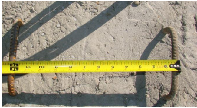
Figure 3-7 Spacing of horizontal shear reinforcement
