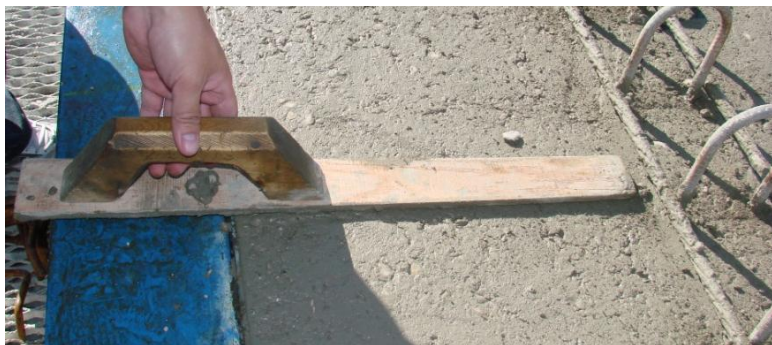
Figure 3-9 Application of wood float finish
