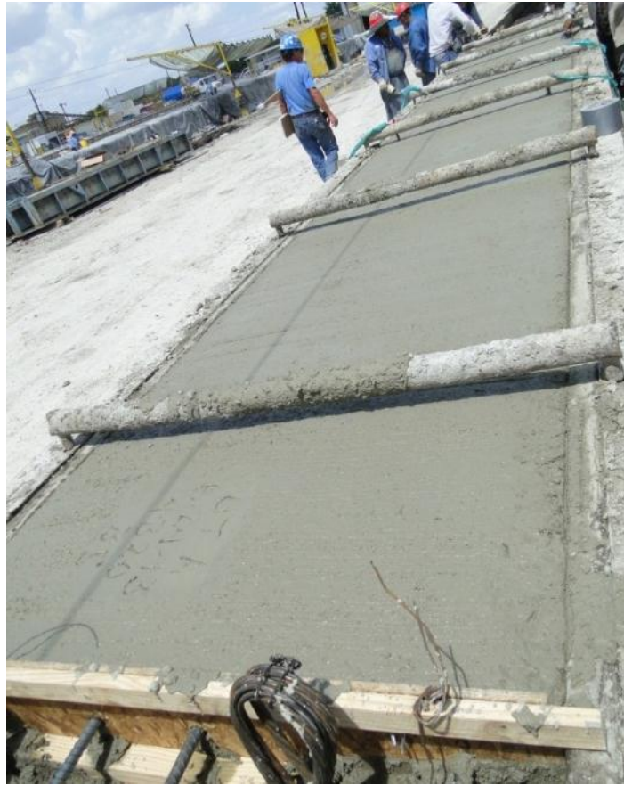
Figure 4-48 Finished box beam after casting
