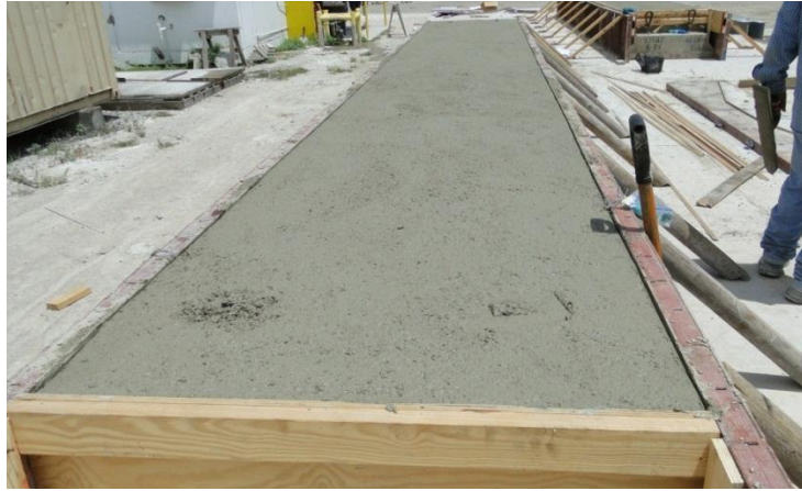
Figure 4-67 Finished box beam specimens
