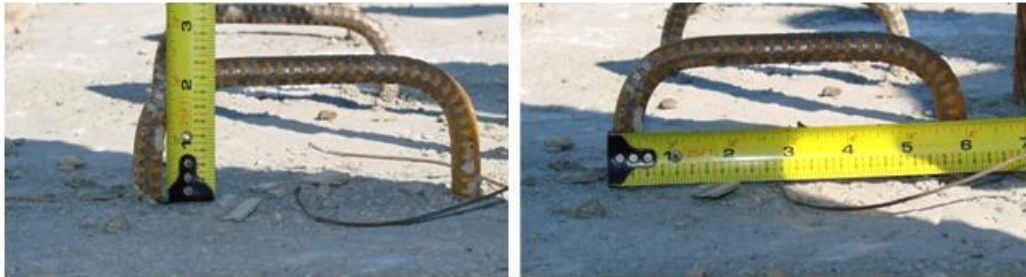
Figure 3-8 Horizontal shear reinforcement details
