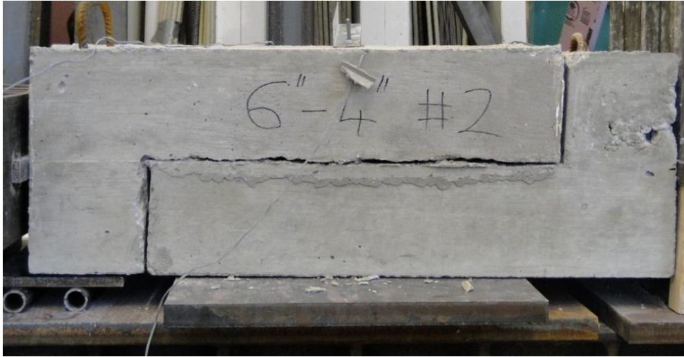
Figure 5-6 Typical failure mode of push-off specimen failure with a 4-in. embedment; no pullout of the bar was observed
