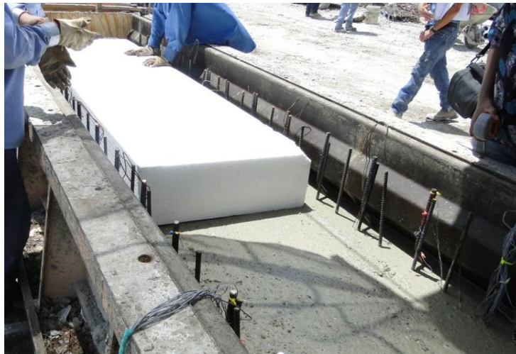
Figure 4-43 Placing of the Styrofoam
