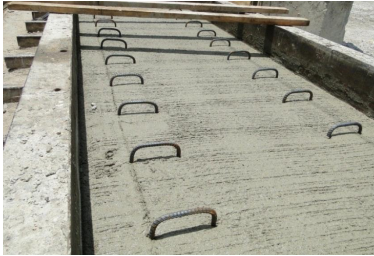
Figure 4-55 Finished slab beam with horizontal shear reinforcement
