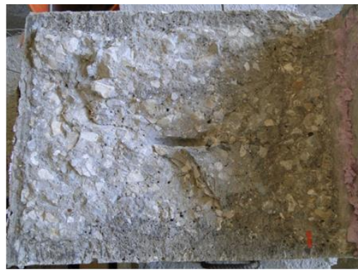
CIP slab failure plane
