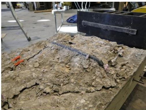
Precast failure plane
