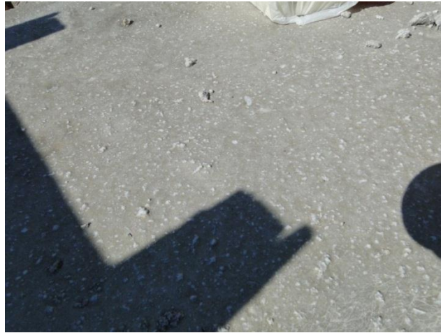
Figure 4-87 Surface finish on SCC slab beam
