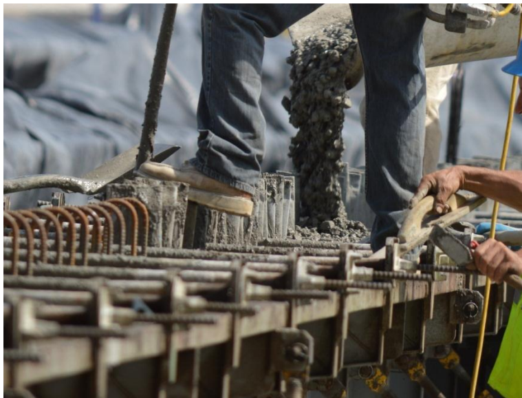
Figure 3-18 Wood float finish provided
