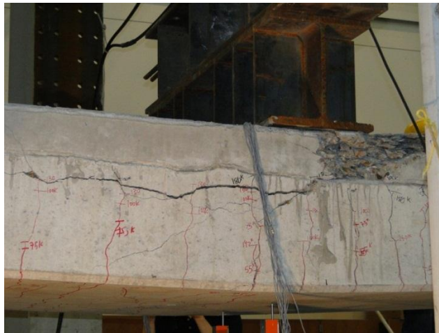
Figure 5-18 Failure at north-face side
