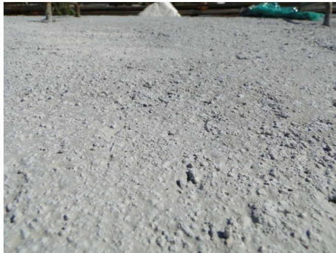
Figure 4-78 Surface finish on box beam
