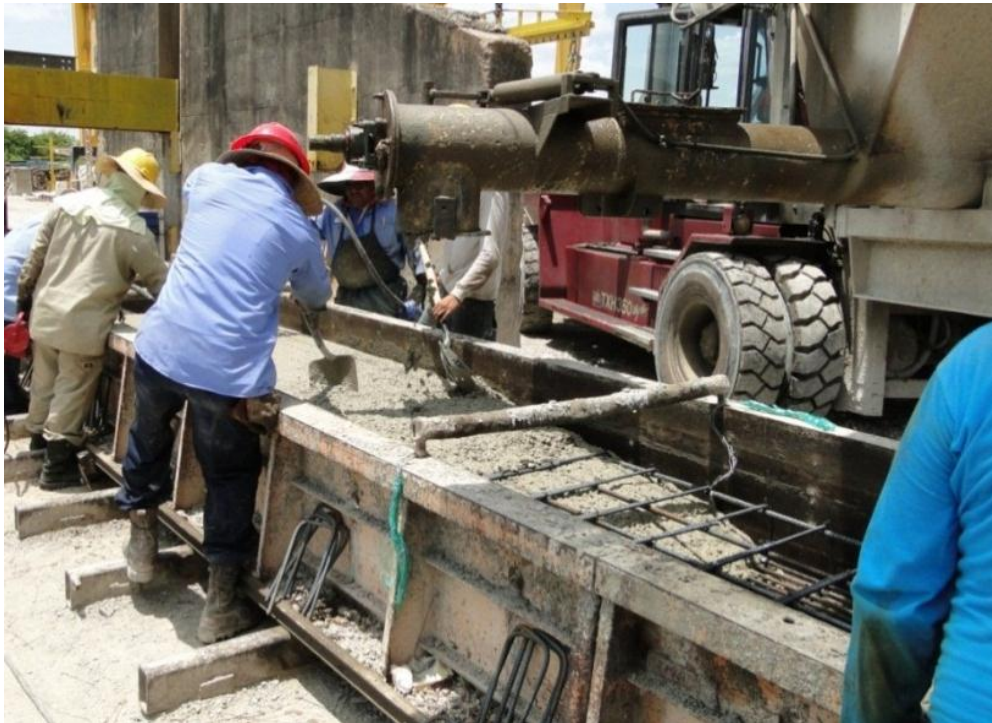
Figure 4-52 Slab beam casting
