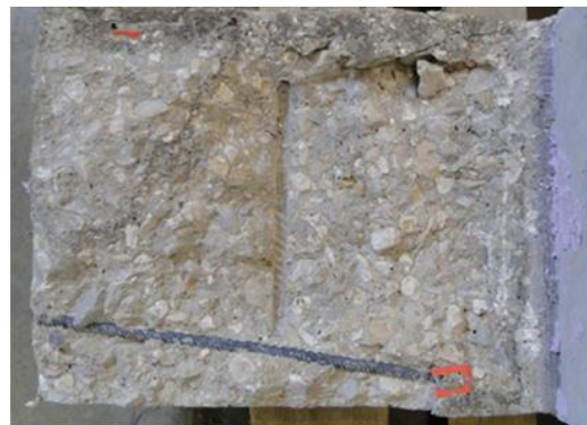
CIP slab failure plane
