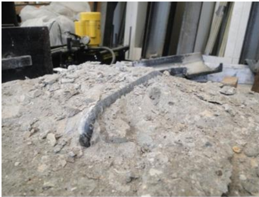
Precast failure plane
