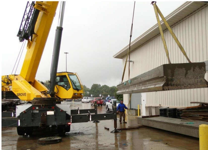
Figure 4-70 Unloading of box beams
