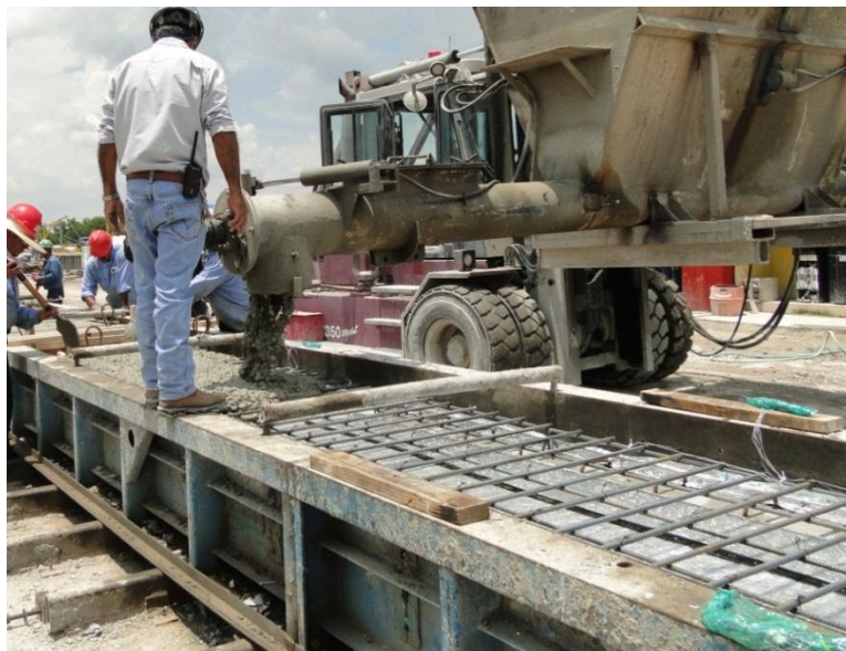
Figure 4-95 Casting of CIP slab
