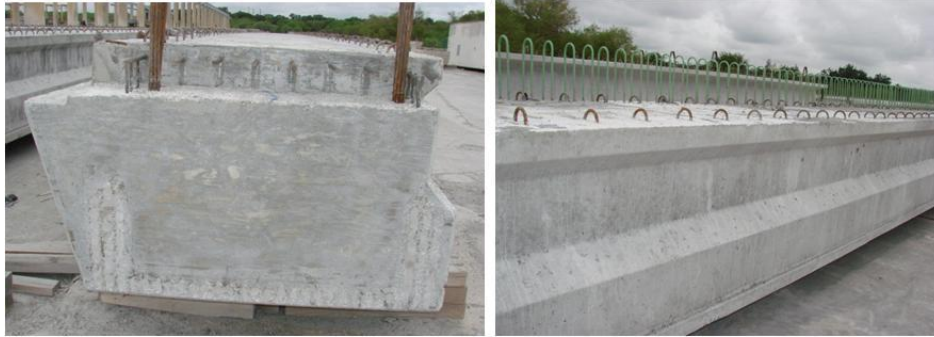
Figure 3-12 Finished box beam
