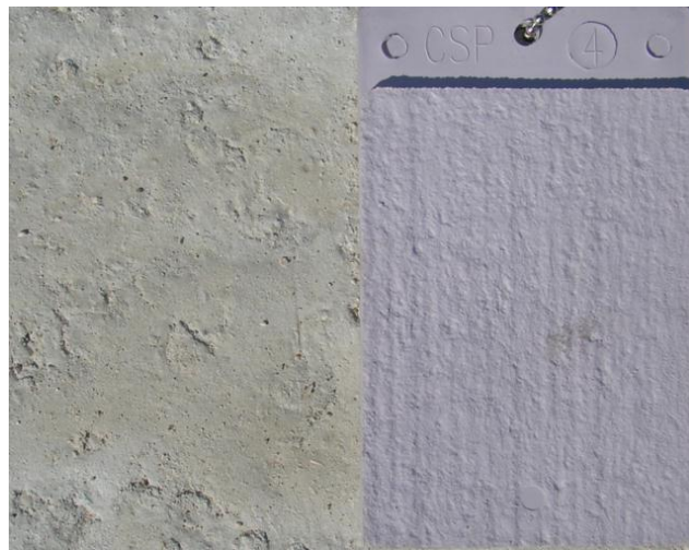
Figure 4-15 Surface finish on SCC slab beams comparable to CSP 4
