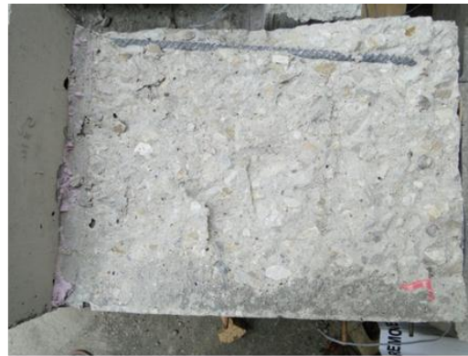
CIP slab failure plane
