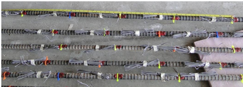
Figure 4-73 Strain gauges on longitudinal reinforcement
