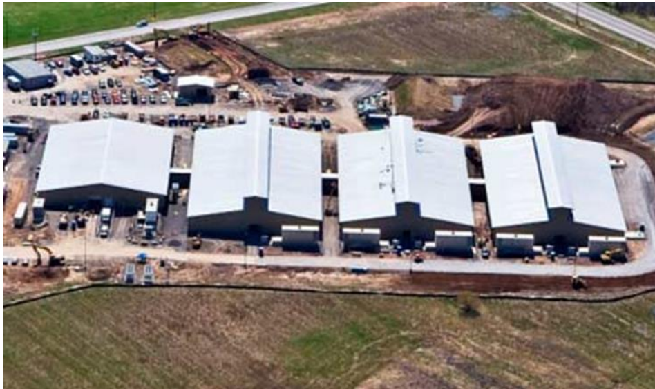
Figure 2 Yahoo Compute Coop Data Center facility[5]
