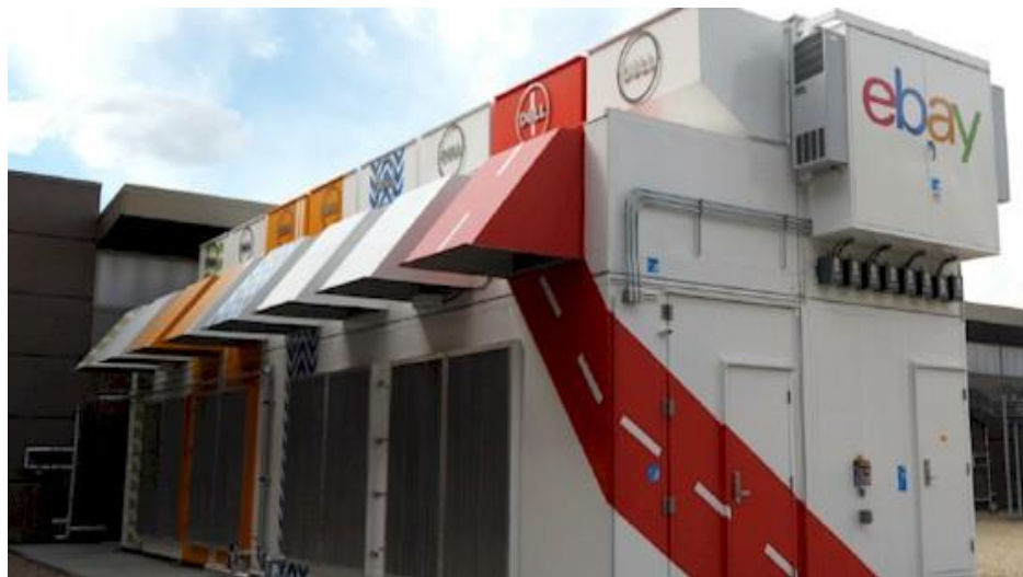
Figure 1 Dell EPIC Modular Data Center for eBay [4]
