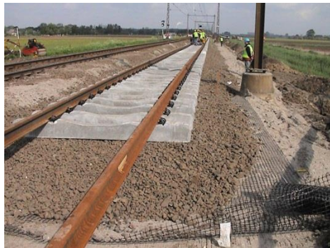
Figure 2-21 Geogrid reinforcement of railway ballast (Tensar 2015)
