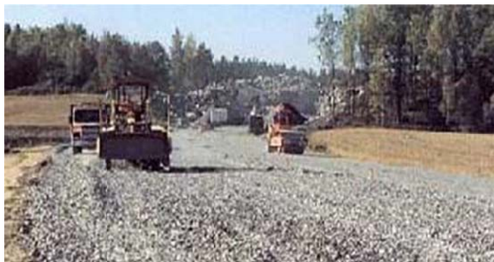
Figure 2-4 Asphalt pavement granular sub-base course
