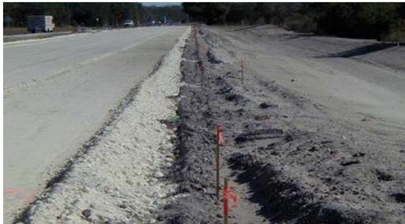
Figure 2-3 Asphalt pavement base construction (Photo by NCAT)
