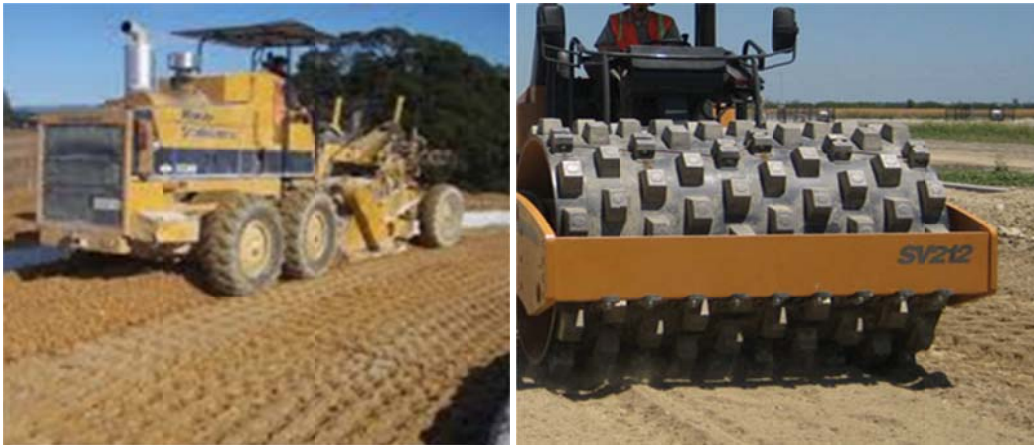
Figure 2-5 Subgrade Construction
