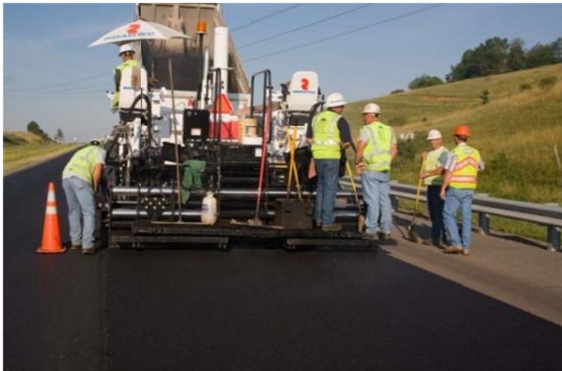
Figure 2-2 Flexible pavement wearing course construction (courtesy of RODTEC)
