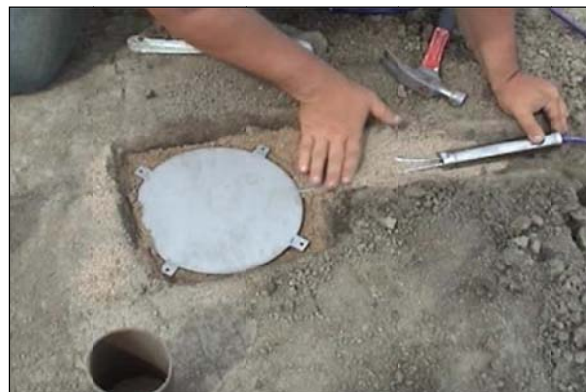
Figure 3-9 Geokon Stress Cell
