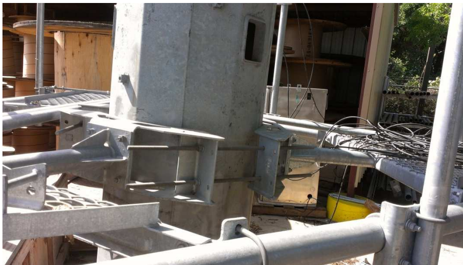
Figure 1.12 Tower leg connectors
