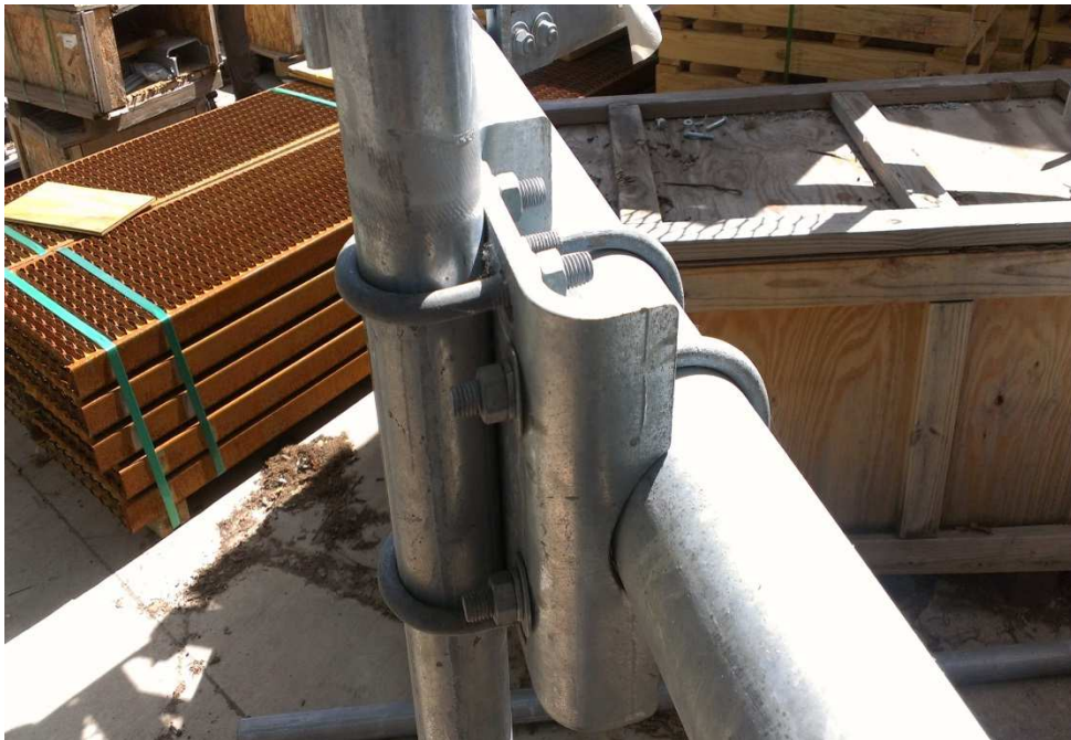
Figure 1.10 Connector plates and bolts
