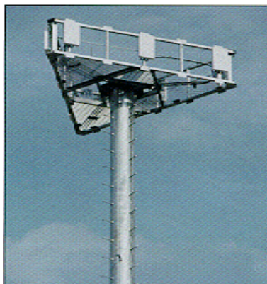
Figure 1.2 Monopole Tower [13]
