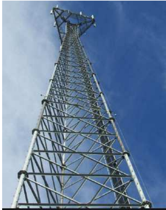
Figure 1.3 Self-supporting Tower [13]
