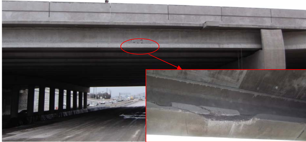
Figure 1-3 Damaged Girder
