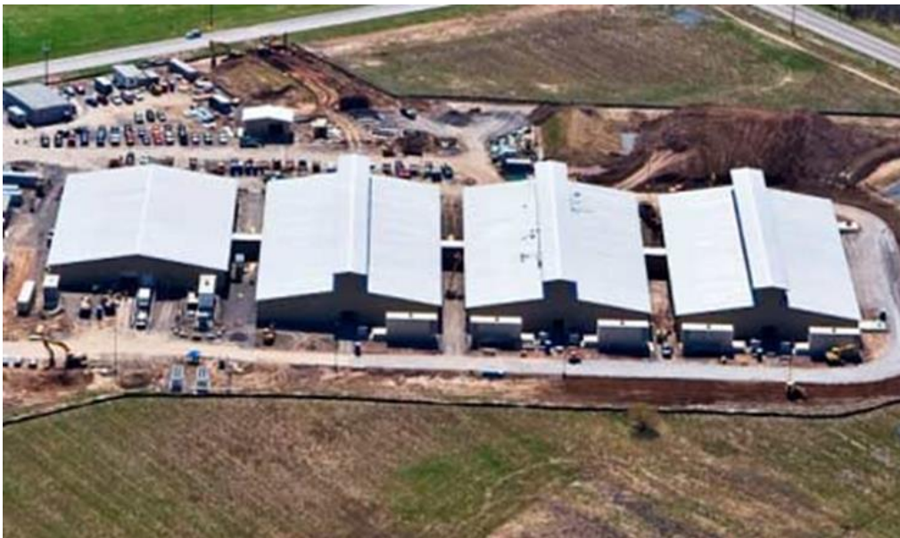
Figure 2: Yahoo Compute Coop Data Center Facility
