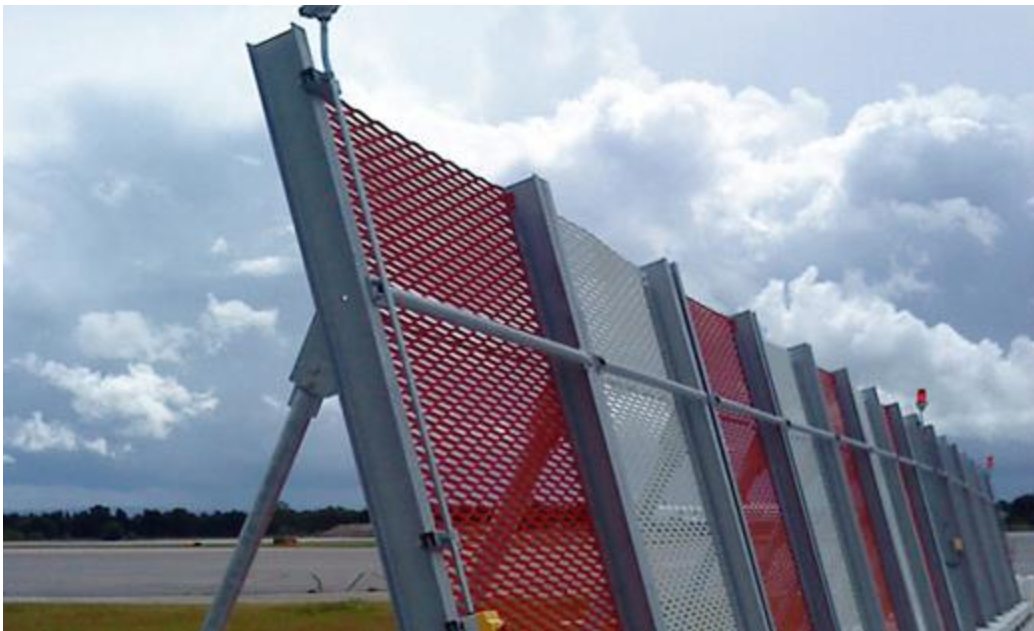
Figure 3: Wind fences used at airports 2
