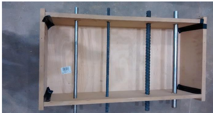
Figure 3-6: Formwork and placement of rebars
