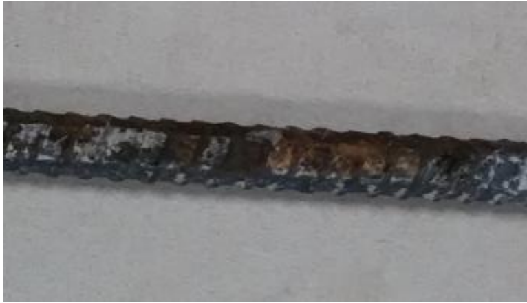
(a) Rebar before cleaning
