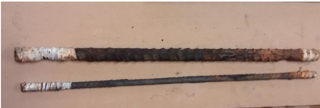
(a) Rebars before cleaning
