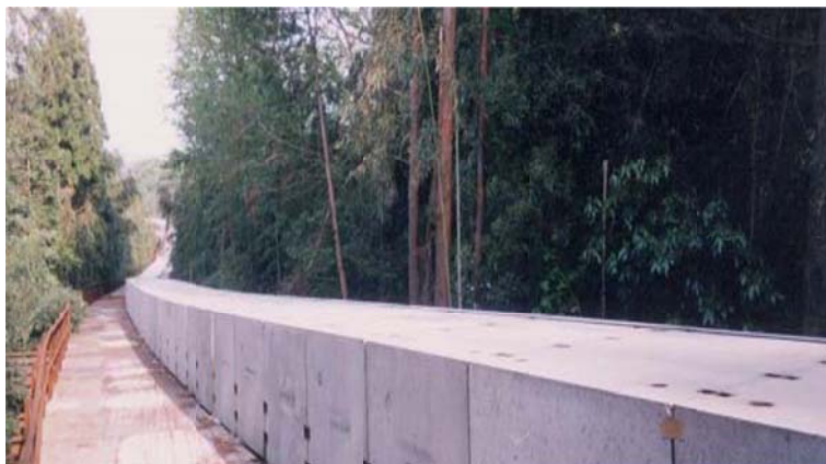
Figure 3.3 PCP extending outside the tunnel to the dump site (Source: Liu, 2004)
