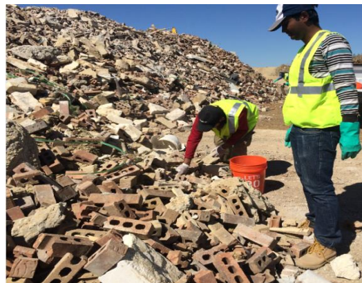
Figure 3.2 Collection of C&D waste samples
