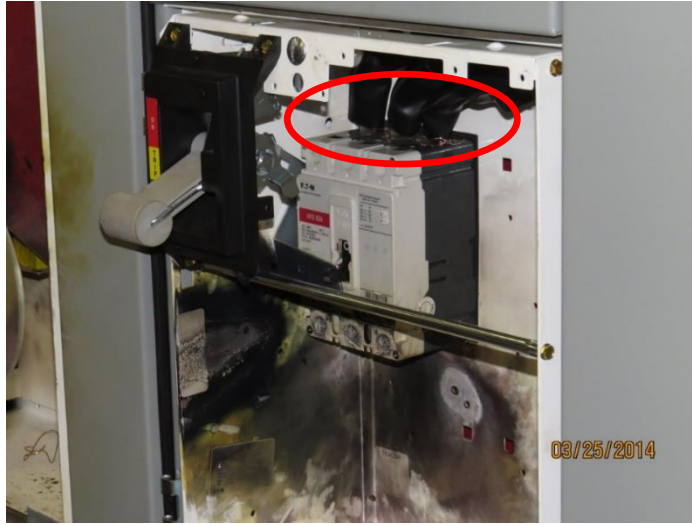
Figure 4- 38 VCBB configuration on switchgear
