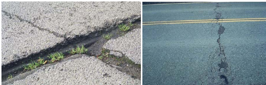
Figure 2. 5: Reflection cracking
