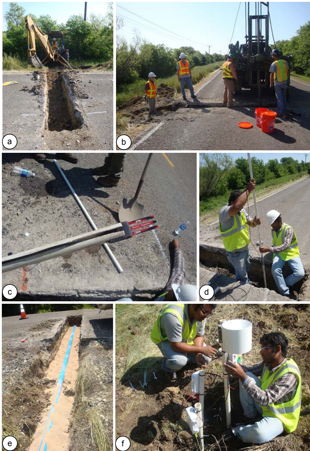
Figure 3. 17: Instrumentation of southbound lane (second stage)
