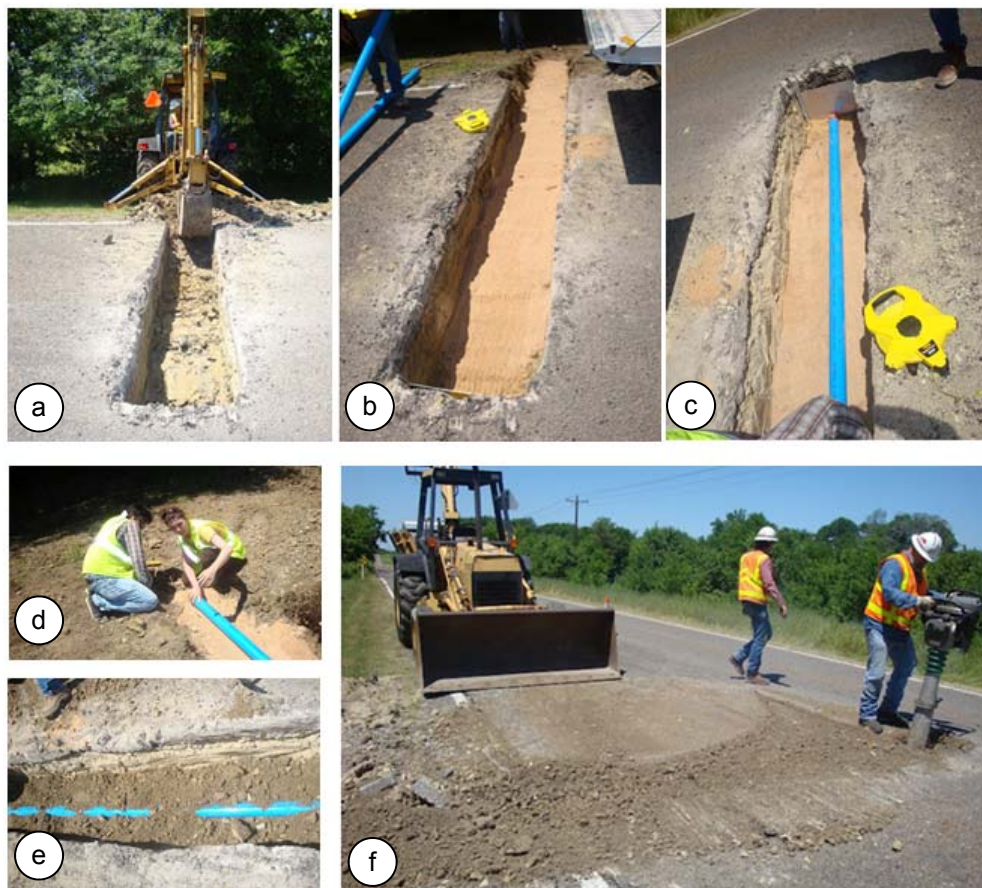
Figure 3. 16: Instrumentation of northbound lane (first stage)
