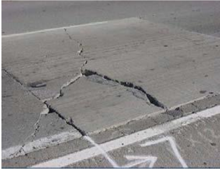
Figure 2-1 Rigid pavement slab cracking (Caltrans, 2008)
