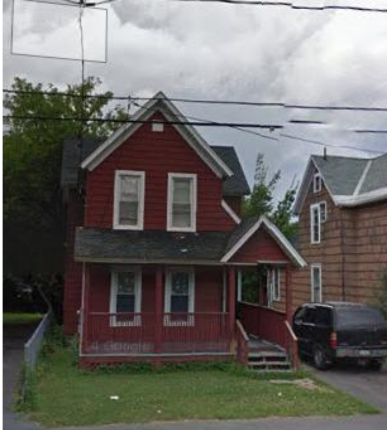
Figure G.1. House L General View
