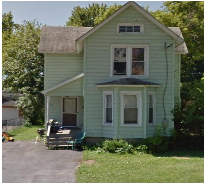
Figure D.1 House E General View
