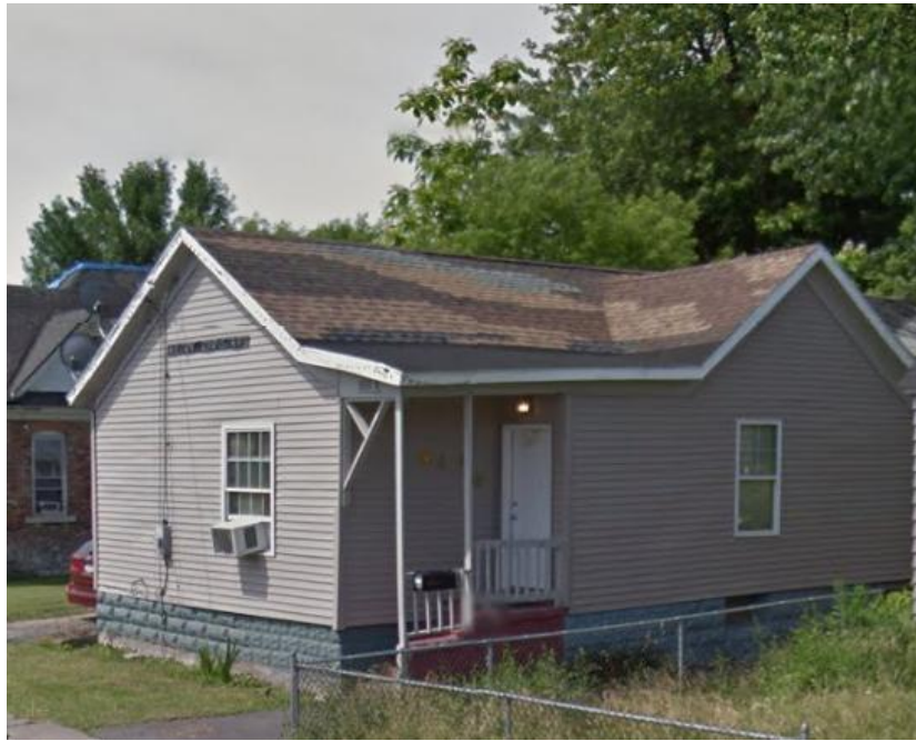
Figure C 1 House C General View
