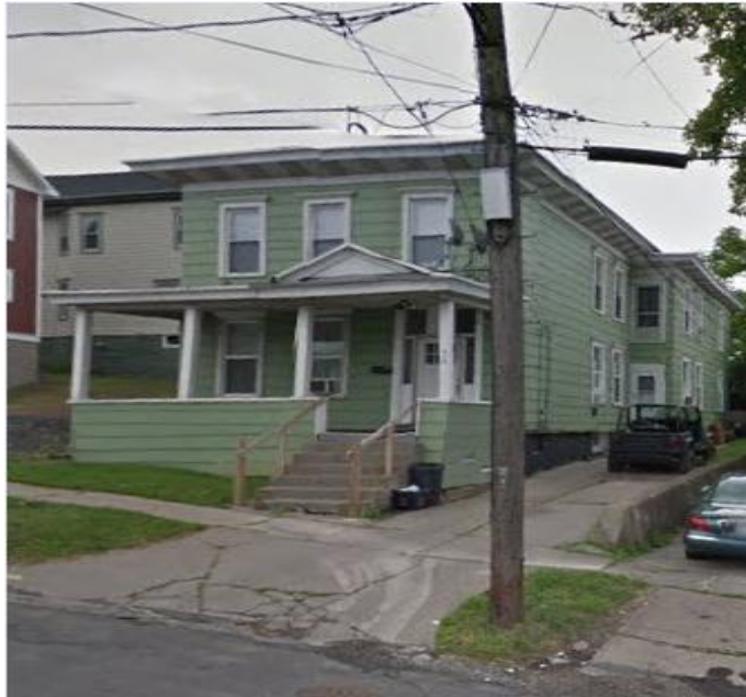
Figure E 1 House J General View
