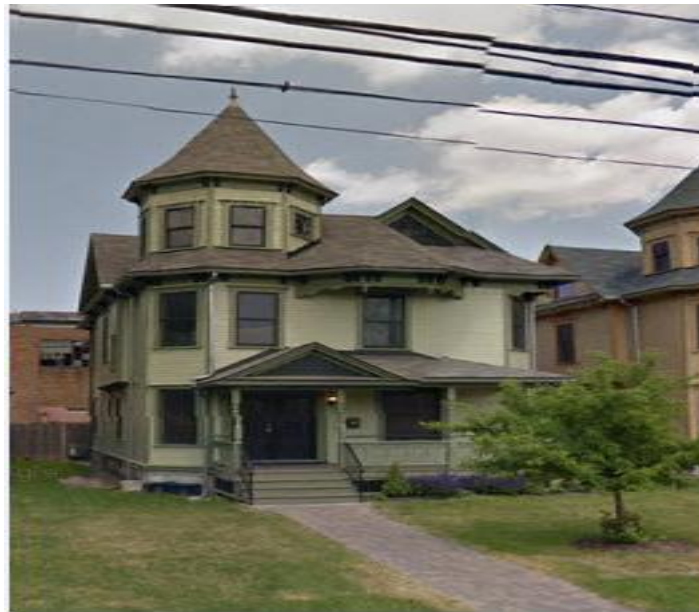
Figure B 2 House B General View
