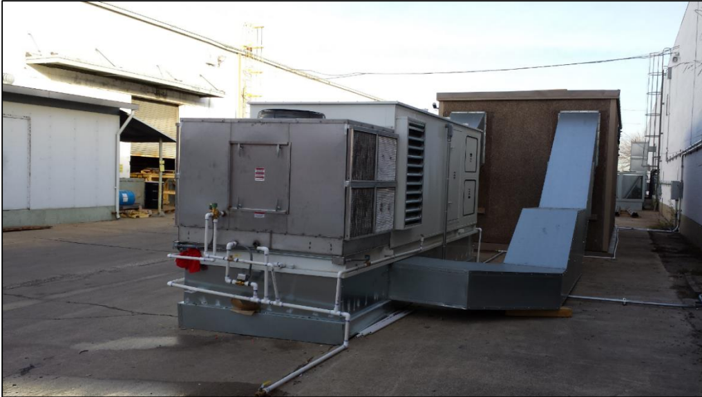
Figure 8. Return Duct Arrangement of Modular Data Center [15]
