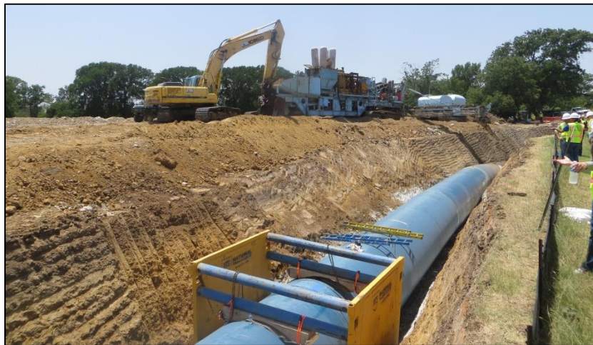
Figure 2-6. Typical Pipeline Installation (Photo by Dr. Najafi)
