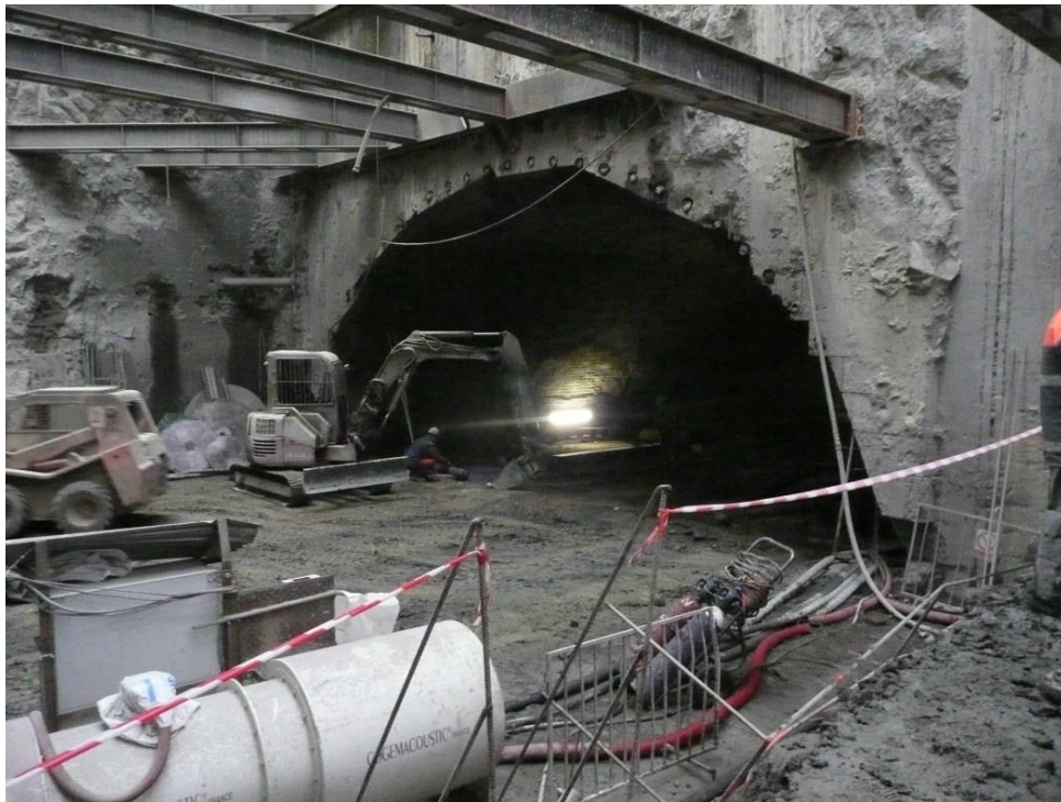
Figure 2-3: Conventional Tunneling in Dobrovského Tunnel, Brno, Czech Republic (Špačková, 2012)
