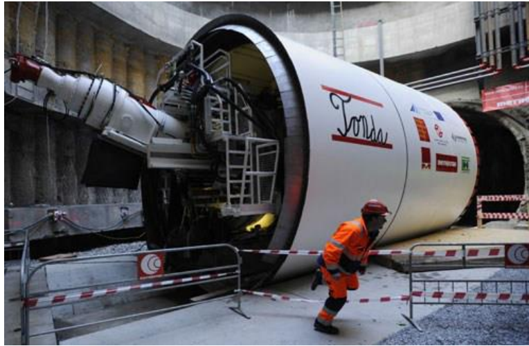
Figure 2-4 TBM Used for Excavation of Underground Line Extension in Prague
