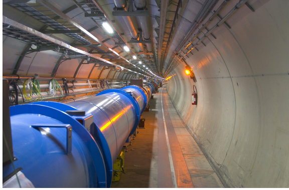
Figure 4.3. A view of the LHC tunnel.
