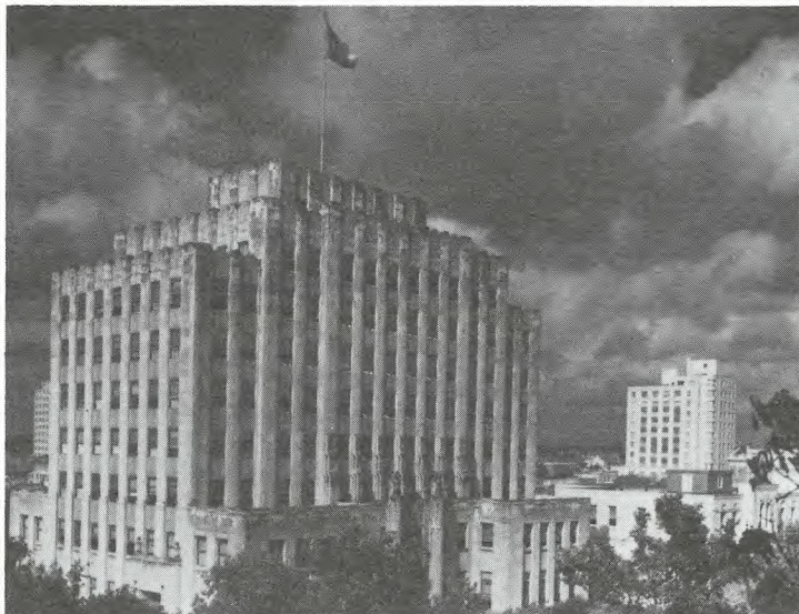
The Registration Division's third home, and home of the Motor Vehicle Division's administrative activities until July 9, 1955, the Highway Building (now the DeWitt C. Greer Building). The white building next to the Highway Building (right) is the former Travis County Courthouse, in use as such until 1930. The building was later used to house state offices.
