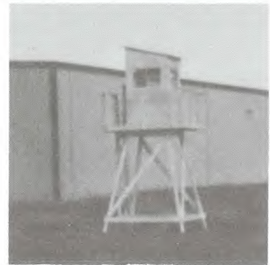
The lonesome picket on the southeast side of the Conversion Building that housed an armed guard.
