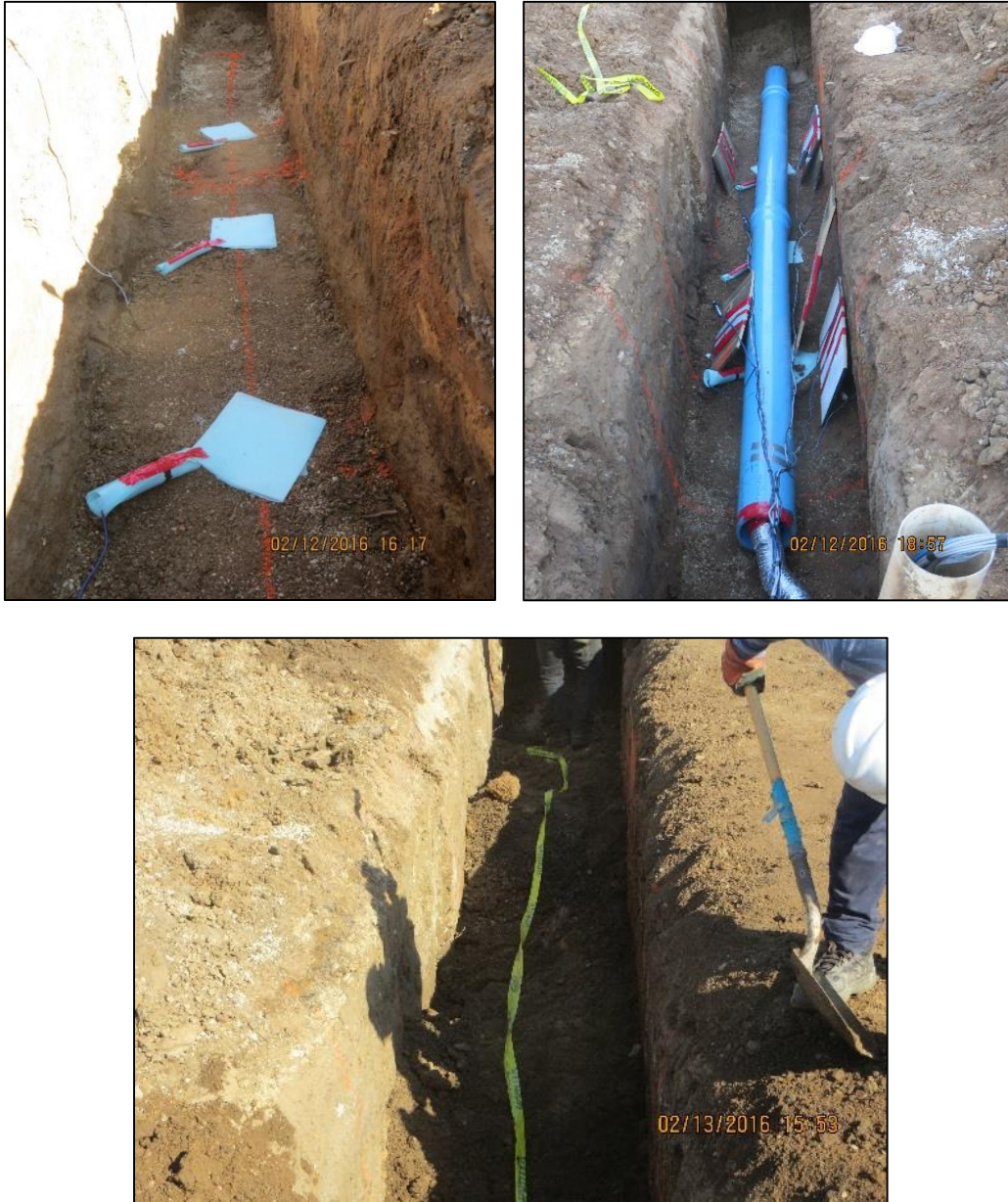
Figure 3-15 iPVC Pipe Installation
