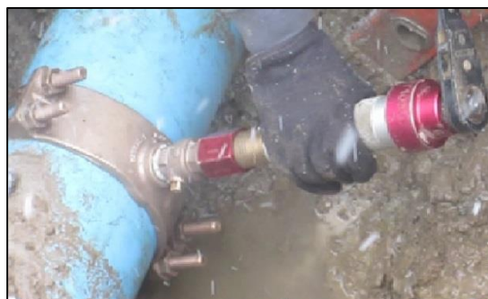
Figure 4-25 Tapping of iPVC pipe (Source: AW)
