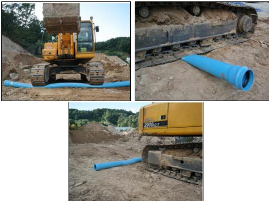
Figure 2-22 Crawl Test (Source: AW and PPI, 2015)
