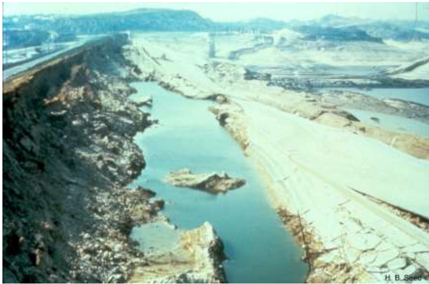
Figure 6.3 Lower San Fernando Dam Failure due to liquefaction in 1971 (Seed, n.d.)
