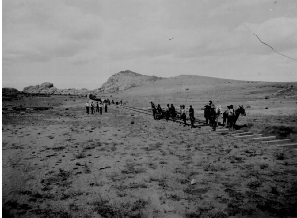
Illustration IV-X: Laying Tracks. 150
