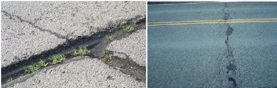
Figure 2:8 Reflection cracking (Hedayati, 2014)
