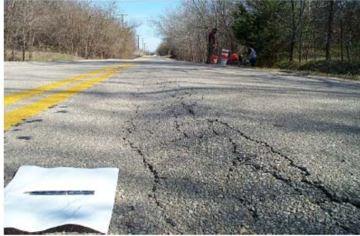
Figure 2:1 Heaving problems in flexible pavements (Manosuthikij, 2008)
