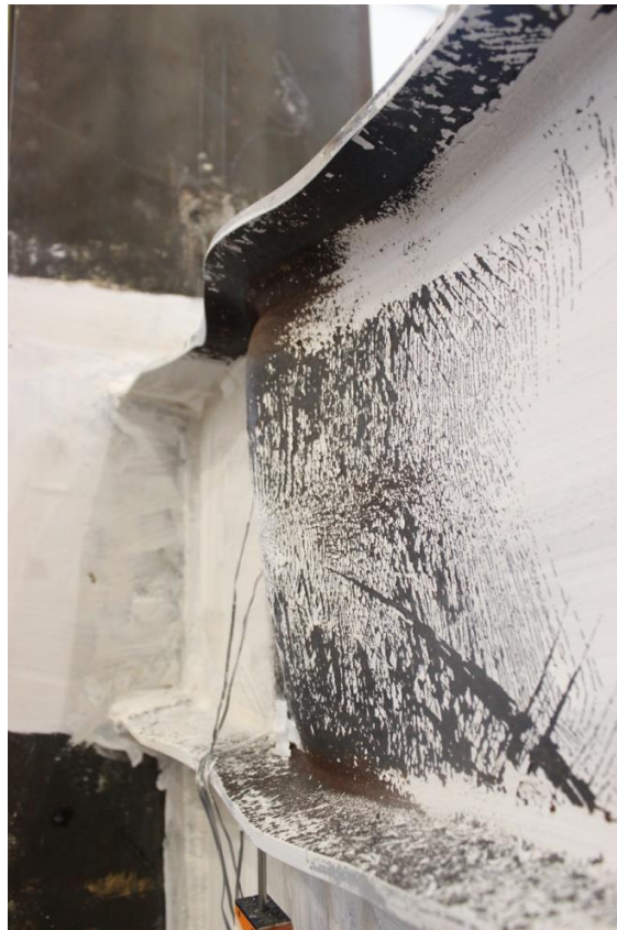
Figure 4-17 Bulging of Individual Channel
