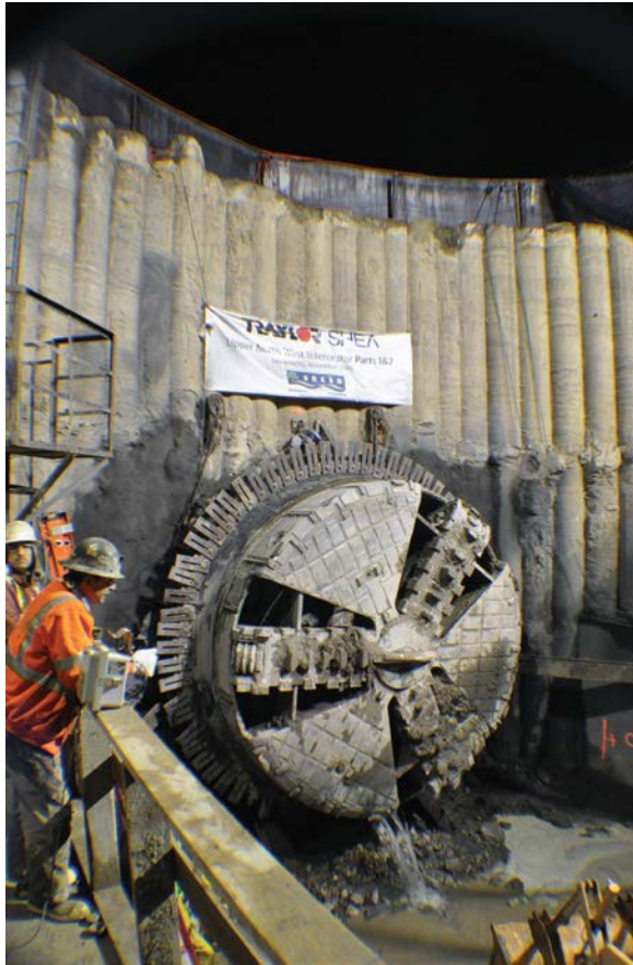
Figure C-12 Breakthrough on November 21, 2009.
