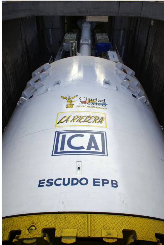
Figure C-5 Robbins 33.5 ft Diameter EPB Excavating Line 12 of Mexico City Metro.
