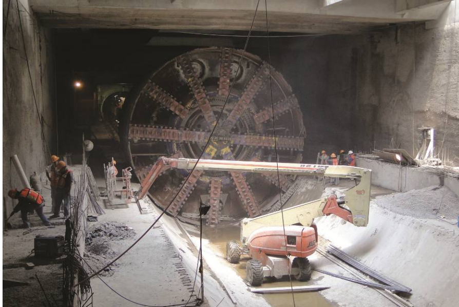
Figure 5-10 TBM Exit into the Ermita Station Robbins Technical Documents, Appendix C
