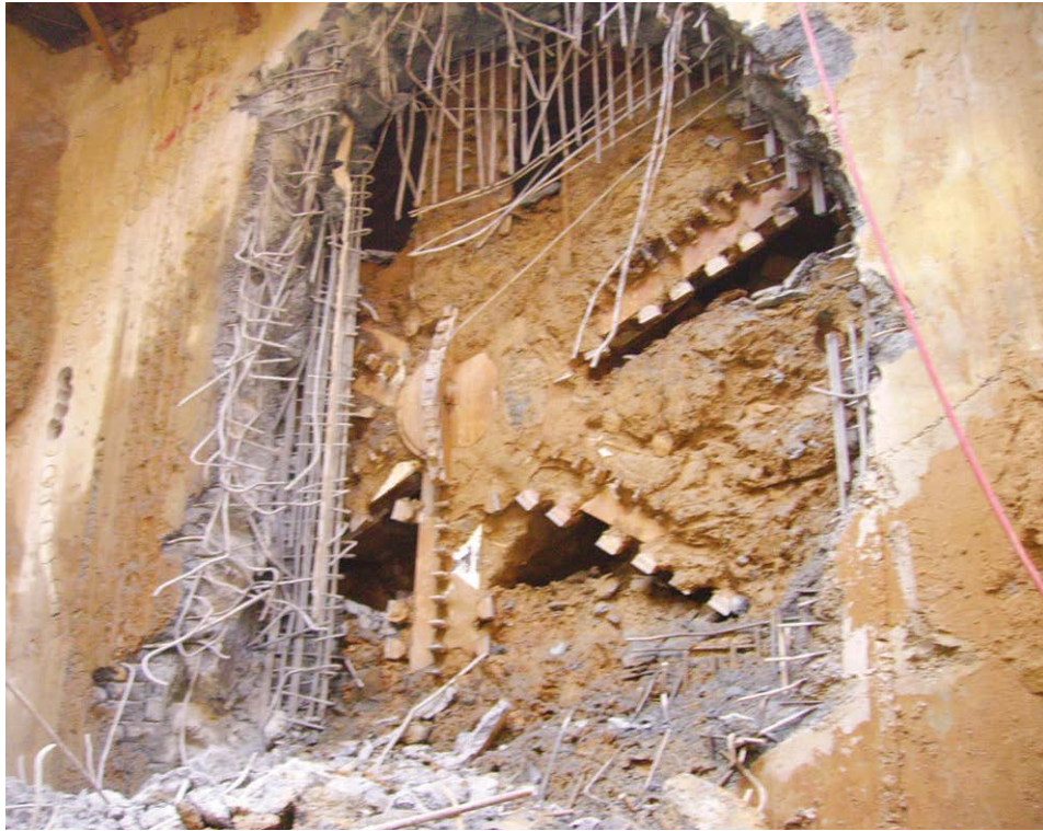
Figure C-11 EPB -324 at its Intermediate Breakthrough in October 2008.
