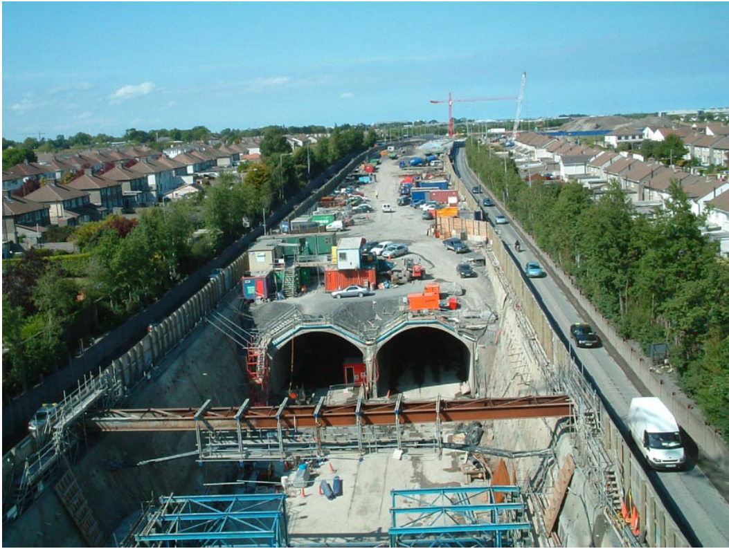
Figure 1-3 Cut and Cover Construction (Tunneltalk, 2017b)
