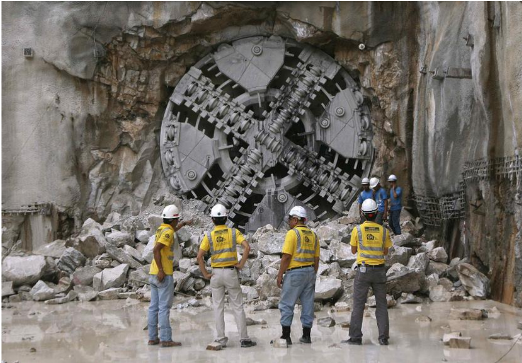
Figure 1-4 TBM at Exit Shaft (Mole, 2017)
