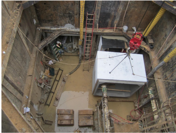
Figure 1-6 Box Jacking Operation (Source: Dr. Najafi, 2017)
