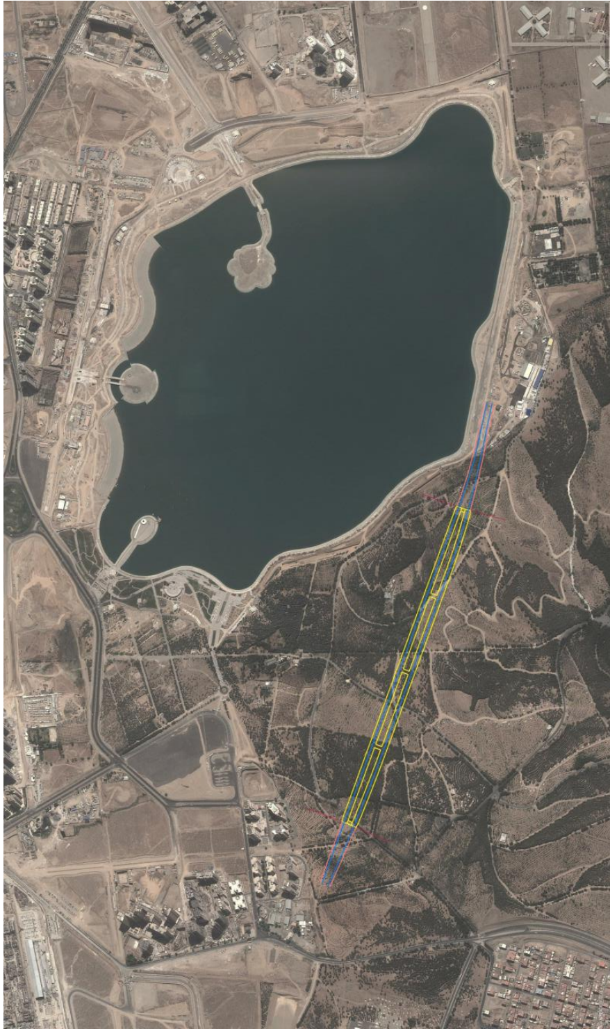
Figure 3-1 Hakim Tunnel Position on a Satellite Image (Google Map)
