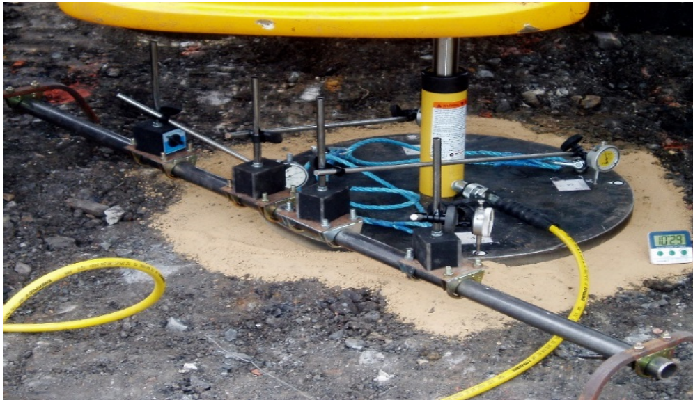
Figure 2-7 In-situ Plate Load Test (Dunelm 2017)
