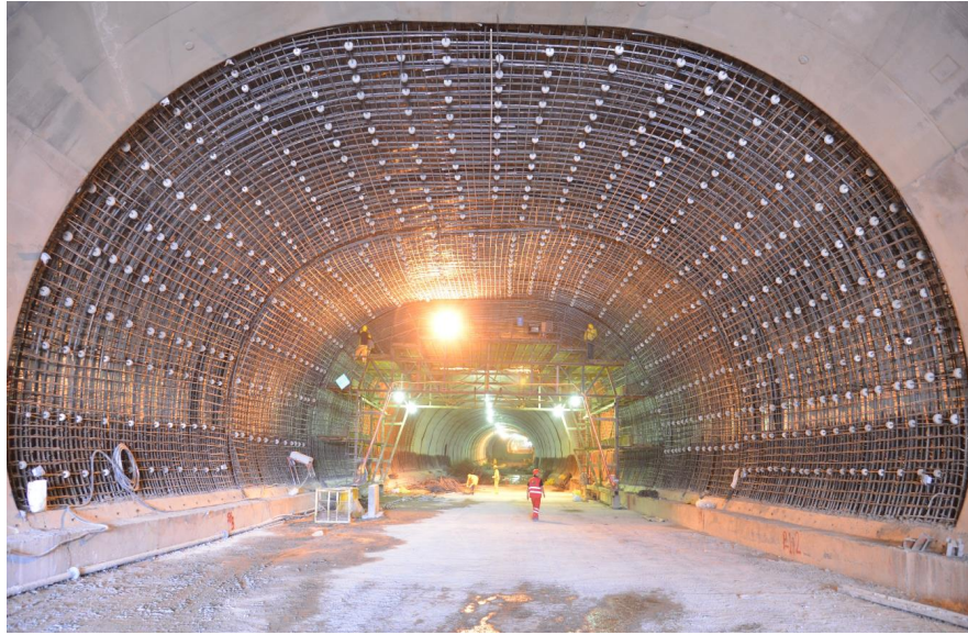
Figure 4-3 Final Lining of Tunnel
