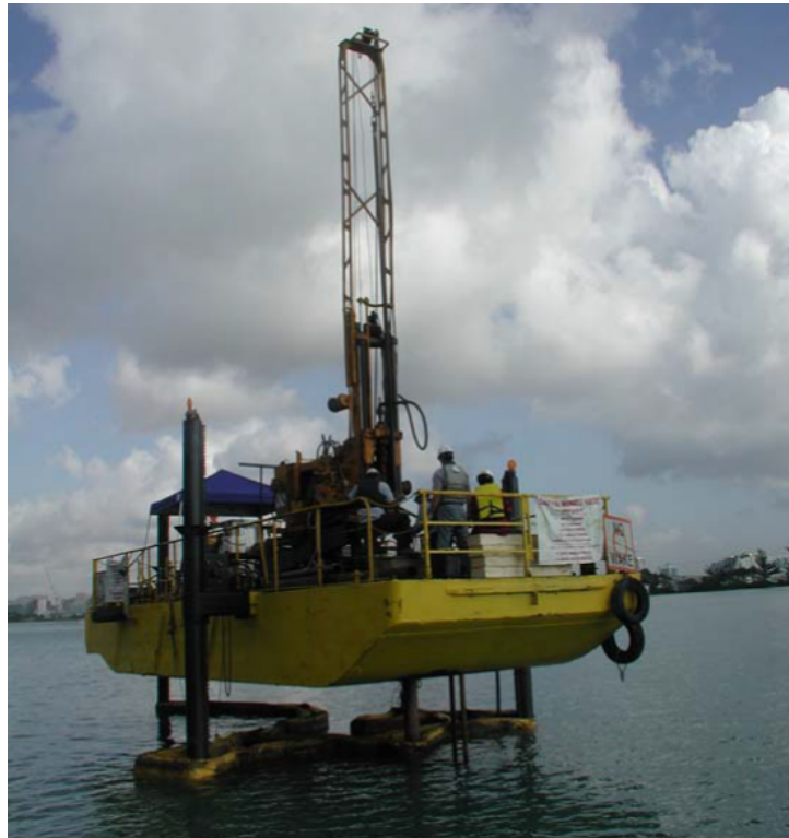
Figure 2-1 Water Boring Investigation in Miami Tunnel (Hung et al. 2009, p. 3-2)
