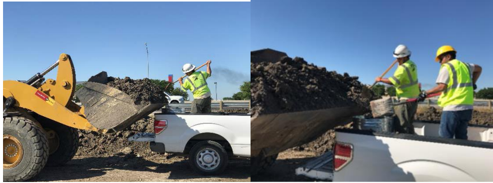
Figure 3-3 Soil sample collection, SH 114, Dallas County
