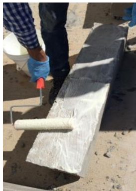
Figure 3 Application of Epoxy
