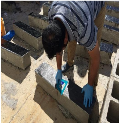
Figure 4 Application of CFRP laminate
