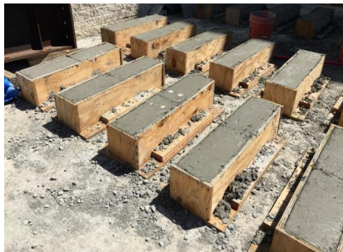
Figure 2 Casting of the beams using ply formwork
