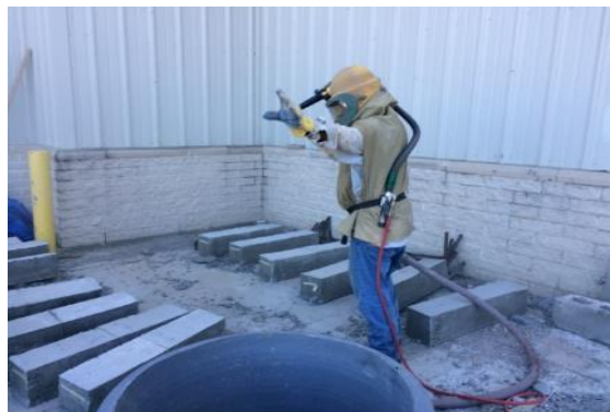
Figure 11 Sand Blasting of Beams
