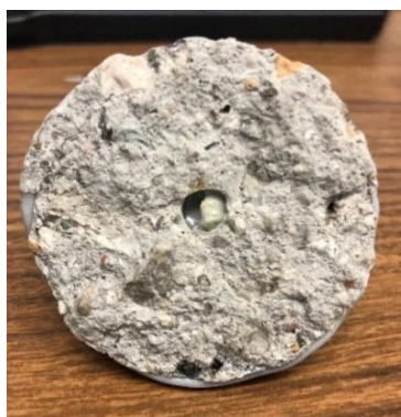
Figure 78 Beam 2, ASTM Pull off test Mode G
