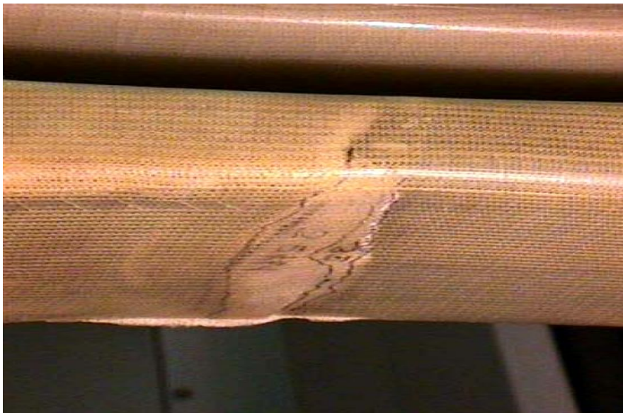
Fig 2.5 Delamination of wrapping layers [1].
