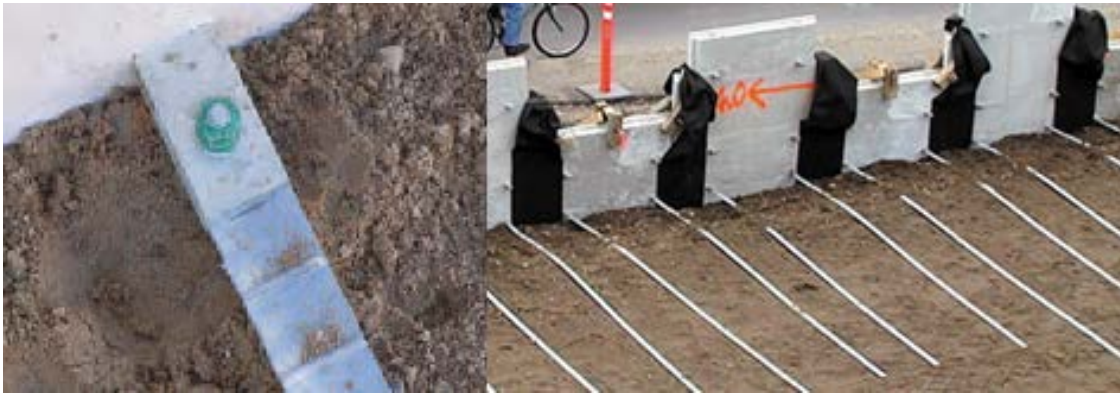
Photograph 2-1 HA Ribbed Soil-Reinforcing Placement (ReCO, 2018)
