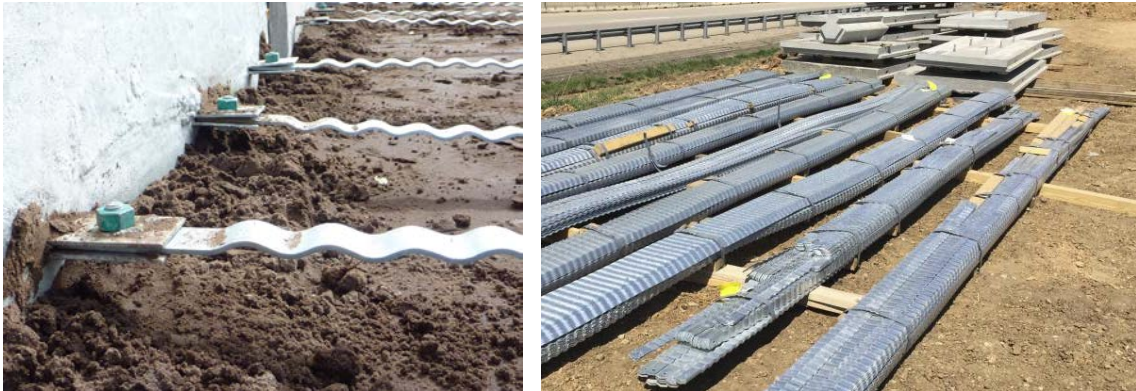
Photograph 2-2 Sinusoidal Soil-Reinforcing Element (Sine Wall, 2018)
