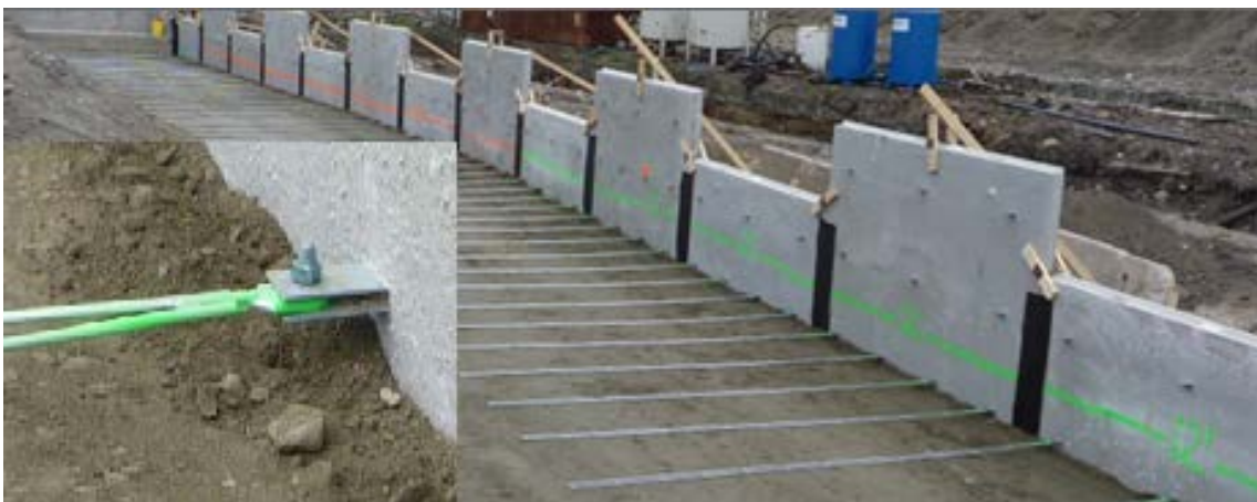
Photograph 2-10 Grid-Strip™ Soil-Reinforcing Placement
