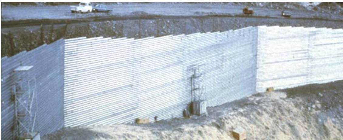
Photograph 1-1 First Reinforced Earth Wall Constructed in United States (NCHRP 1987)
