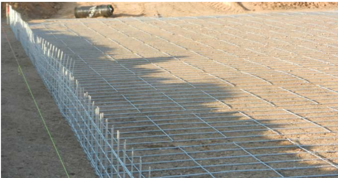
Photograph 2-4 Welded Wire Continuous Coverage
