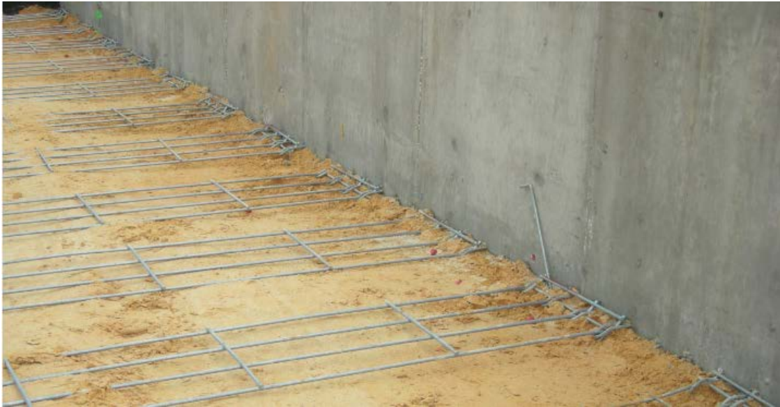
Photograph 2-6 Bar-Mat Soil-Reinforcing Placement
