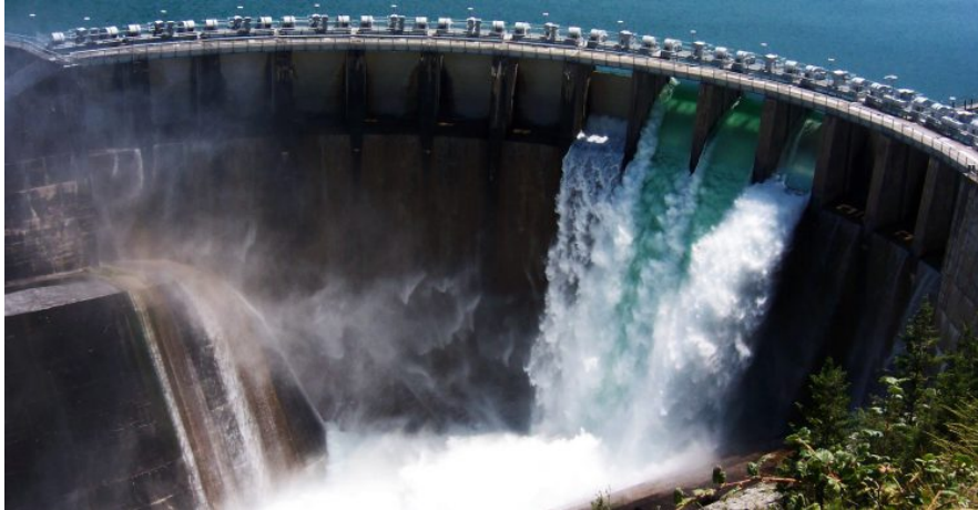
Figure 2.4 Hydropower Dam (Clean Energy Ideas)
