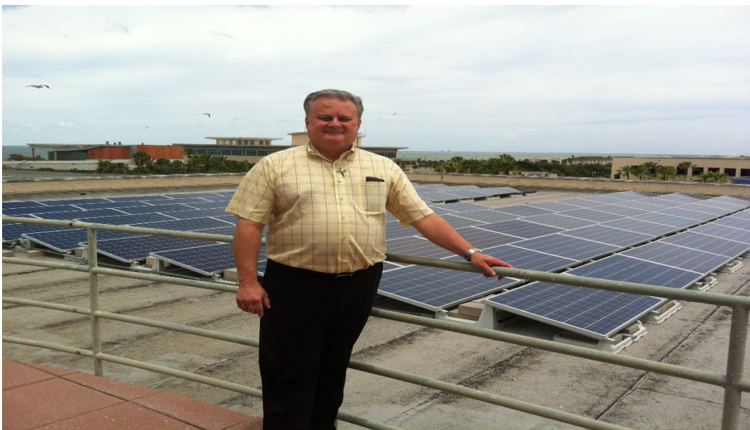
Figure 4.3 Operating Solar Array: Texas A&M University-Corpus Christi
