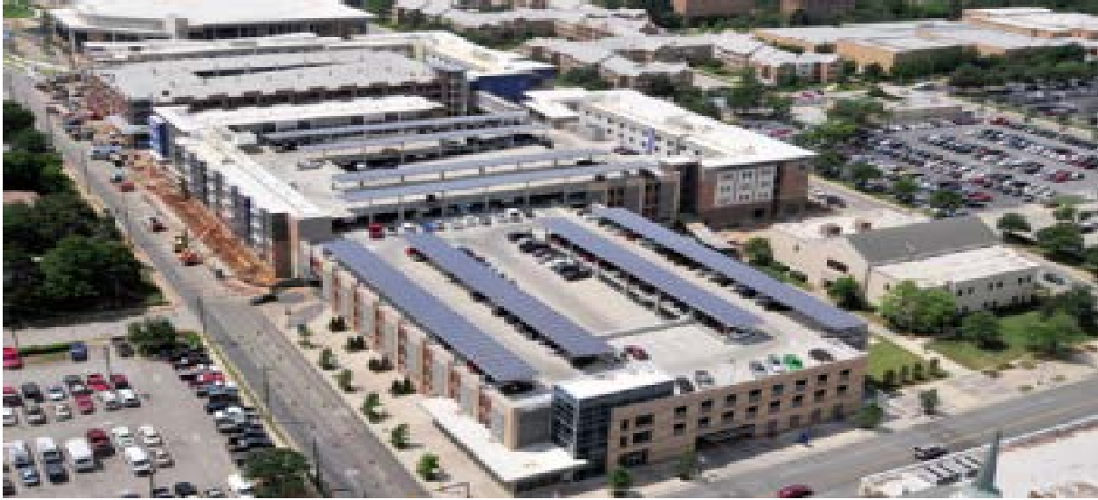
Figure 4.4 Operating Solar Array on Parking Garages: University of Texas at Arlington
