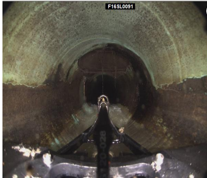
Figure 4-32 Roots intrusion for line 56
