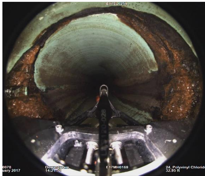
Figure 4-31 Roots intrusion for line 37
