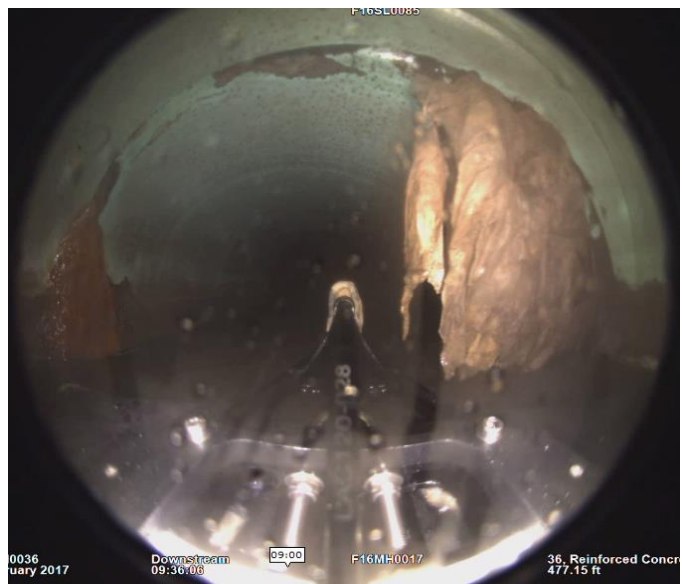
Figure 4-29 Roots intrusion for line 58
