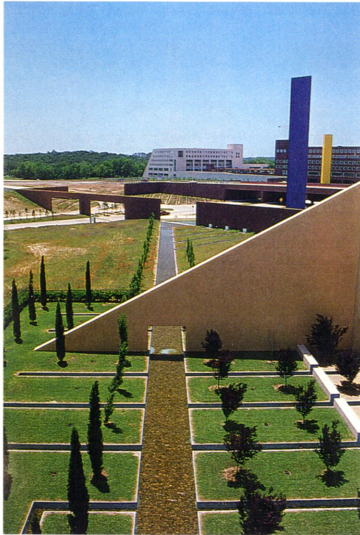
Figure 16. Massive Wing Walls. (Bunji, 1989)
