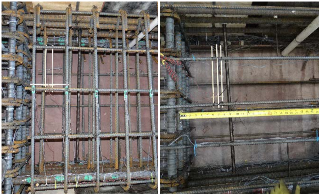
Figure 2.18 Reinforcement in the Joint of HPFRC specimen
