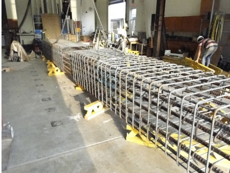
Figure 2.13 Reinforcement cage for beams
