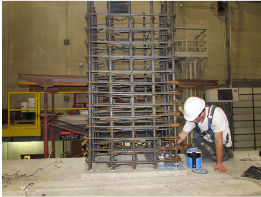
Figure 2.21 Reinforcement cage for top column
