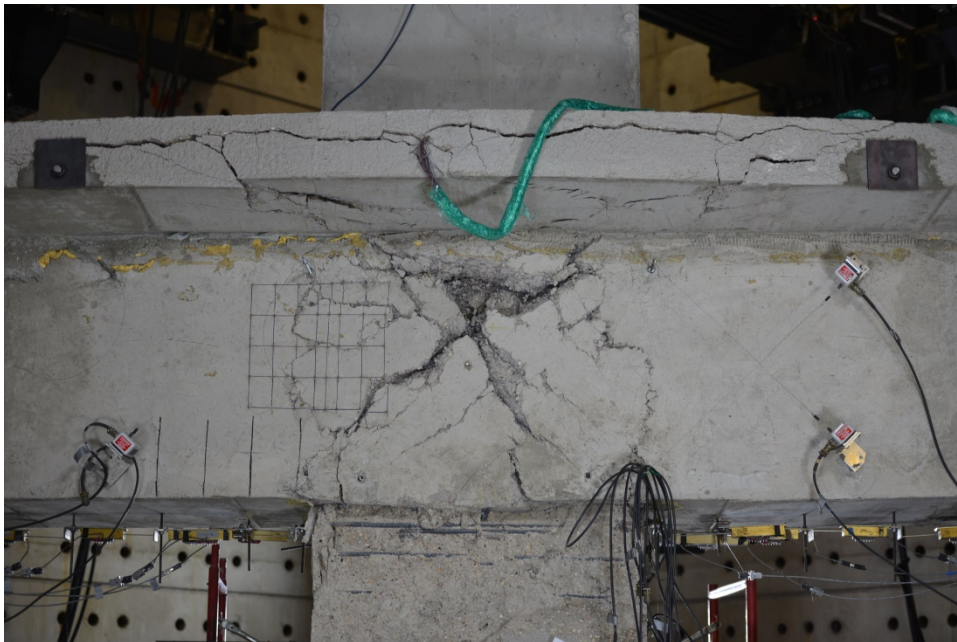
Figure 3.6 Cracks and damage of RC-SP-CL after test
