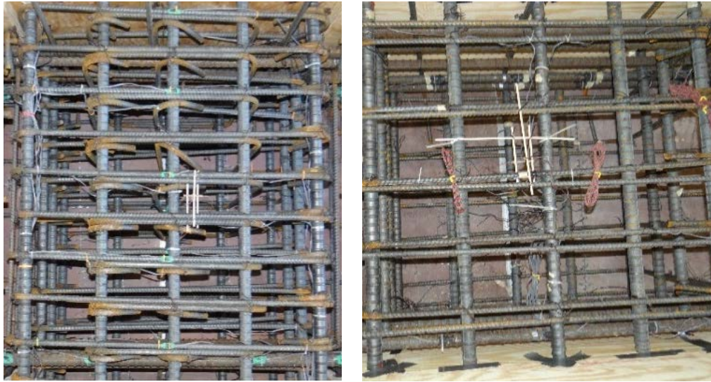
Figure 2.17 Reinforcement in the Joint of RC specimen
