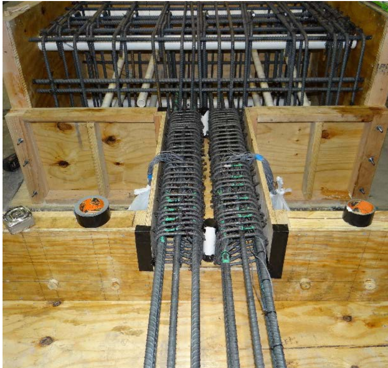
Figure 6.8 Construction photo of DCB
