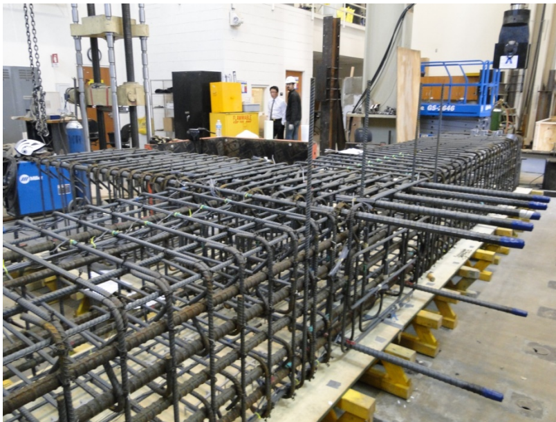
2-16 Final reinforcement cage for beams and lower column
