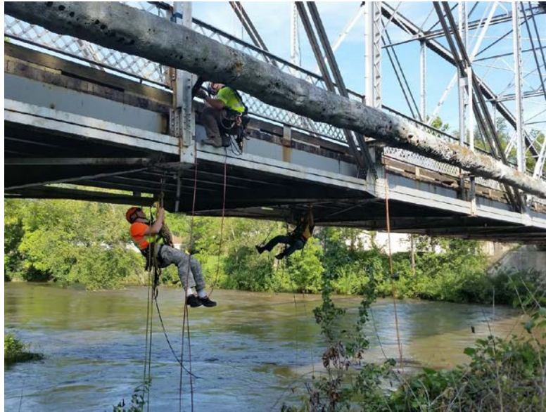
Figure 2-12. Rope Access Inspection (Wells et al. 2017)
