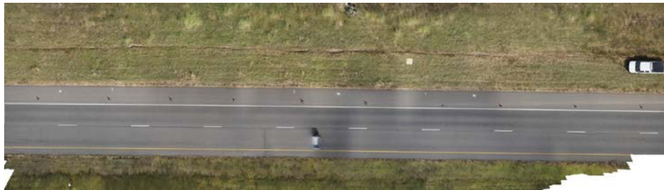
Figure 4-4. Orthomosaic of US 82 Highway Section
