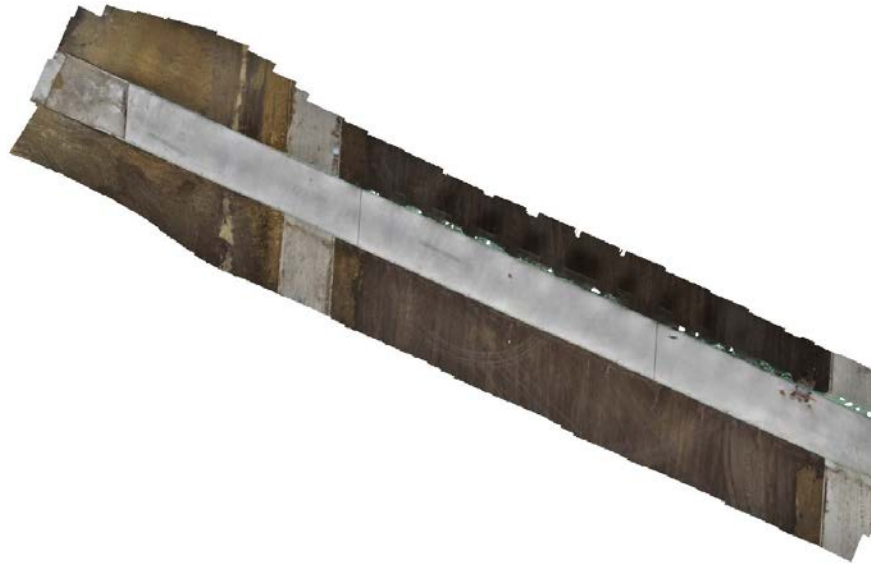
Figure 4-37. Orthomosaic of the Bridge Deck of SH 360 located in Mansfield, Texas
