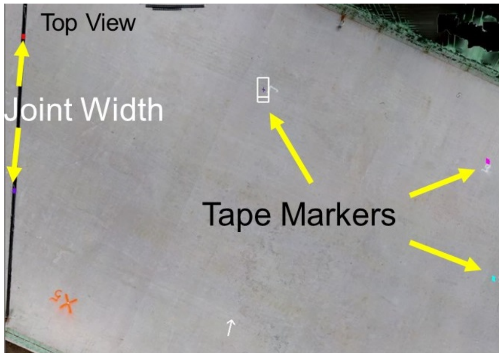
Figure 4-40. Taped Markers and Joint Width Locations on the Bridge Deck
