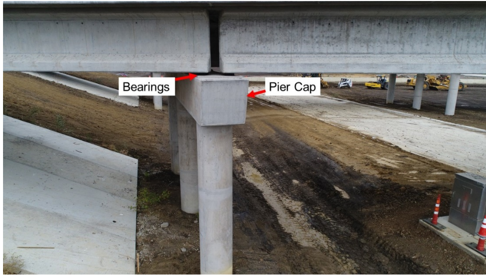
Figure 4-46. Side View of the Bridge Substructure Elements
