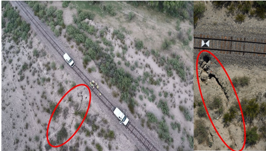
Figure 4-63. Aerial view of Drainage Path That Contributed to the Washout
