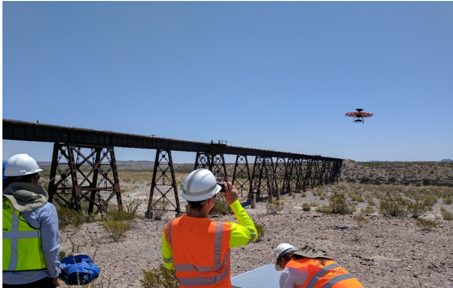
Figure 4-56. UAV with Camera Mounted on Top Gimbal Flying Towards the Bridge for Inspection
