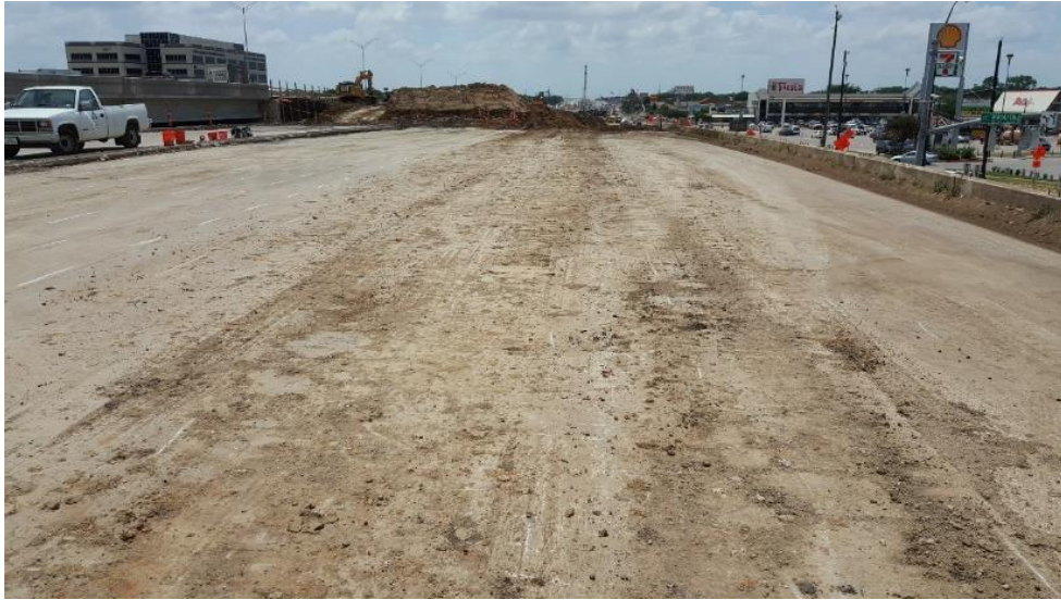
Figure 6-21 Presence of Soil on Deck
