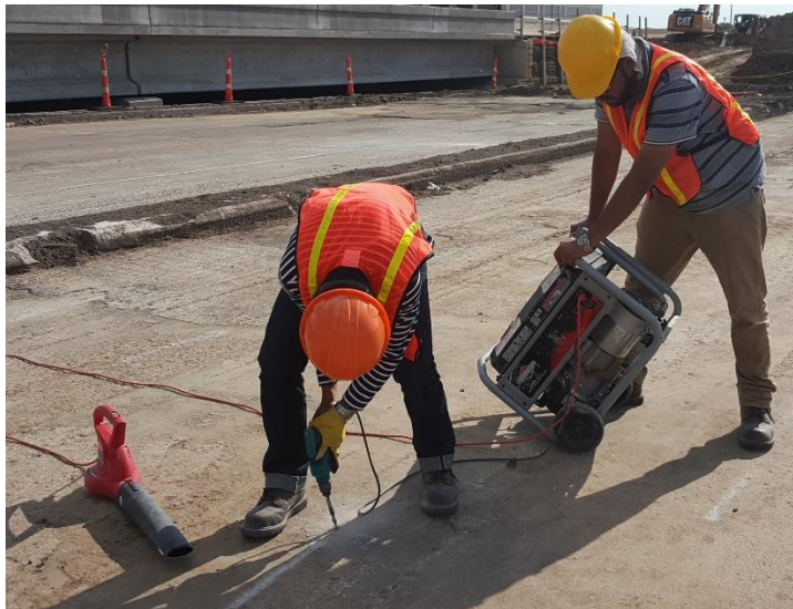
Figure 4-3 Drilling for true concrete cover
