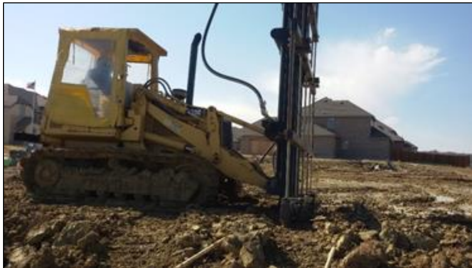
Figure 3-1 Pressure Injection of Ionic Soil Stabilizer in Field
