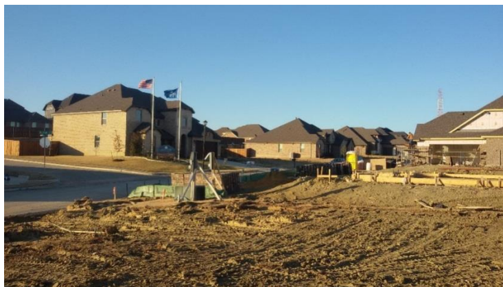
Figure 5-1 Site for soil stabilization
