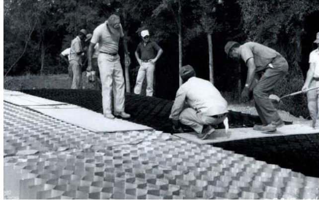
Figure 2.4 Plastic and aluminum cellular confinements used at Waterways Experiment Station, Vicksburg (Source: Presto Geosystems)
