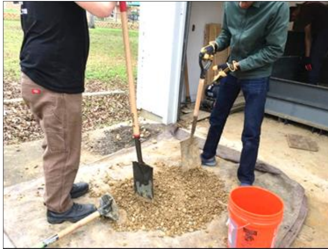
Figure 3.20 Mixing of subgrade material by adding the required moisture content
