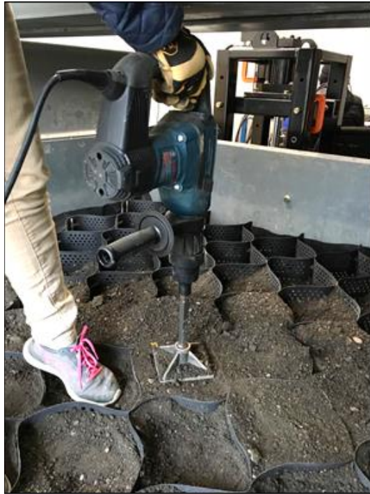
Figure 3.23 Compacting RAP material inside geocell pockets using hand vibratory compactor
