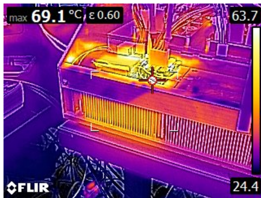
Figure 3.3: One brick operating in burn in station
