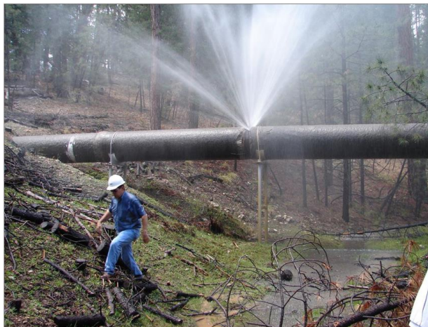
Figure 1-4 Connection failure on Salt River Project that feeds water from the C.C. Craig Dam and Reservoir to the town of Payson Cronkite News Service, Joshua Armstrong
