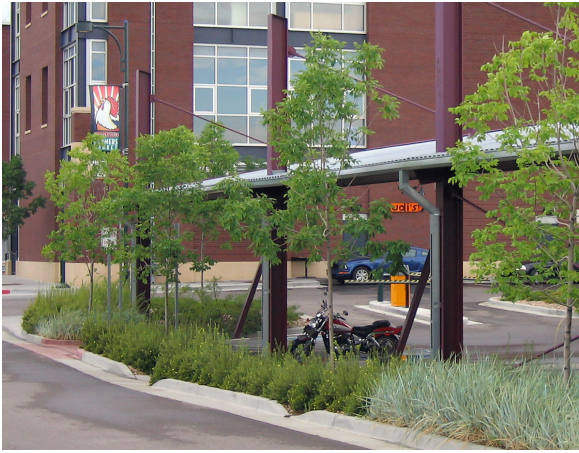
Figure 1 Rain garden in Stapleton Redevelopment, Denver, Colorado
