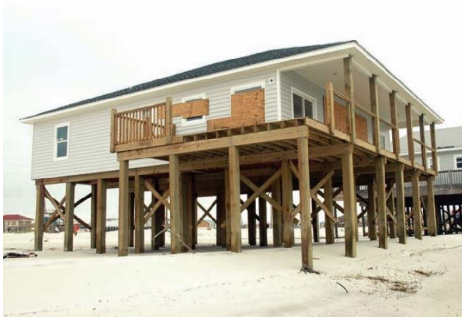
Figure 2.5 Successful pile foundation following Hurricane Katrina (Source: FEMA, 549)
