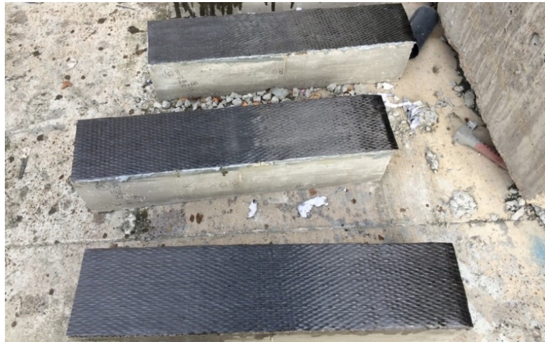
Figure 3-11: The concrete beams after attaching the FRP
