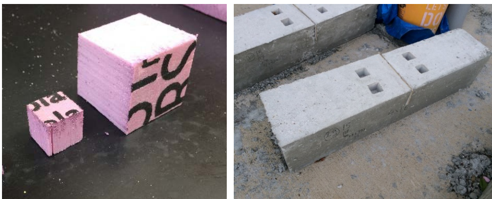
Figure 3-4: Voids preparation
