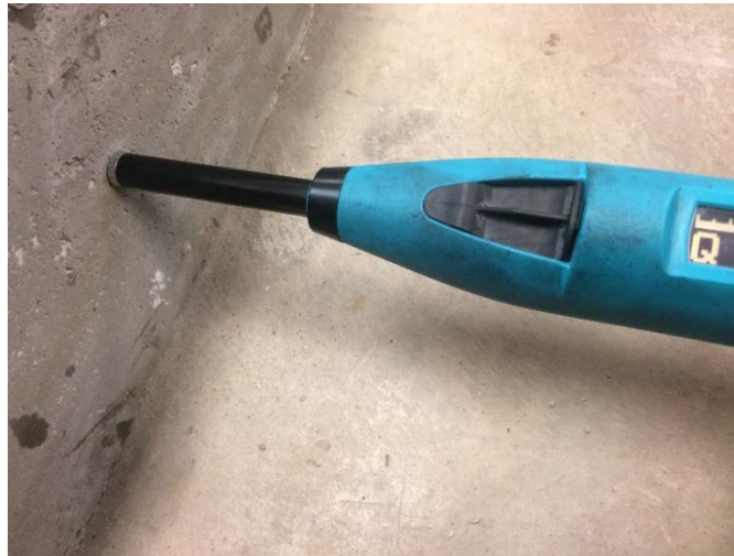
Figure 4- 5: Schmidt hammer testing at the concrete surface
