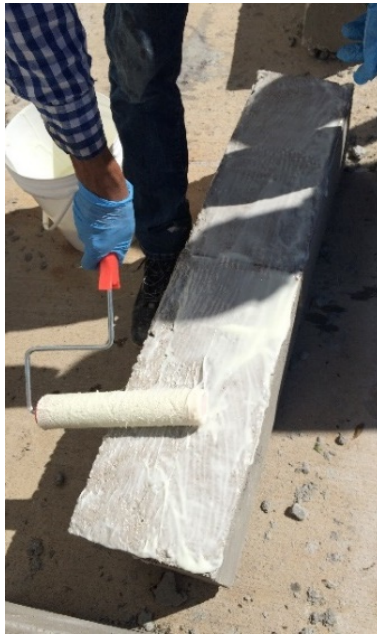
Figure 3-9: Applying the Epoxy
