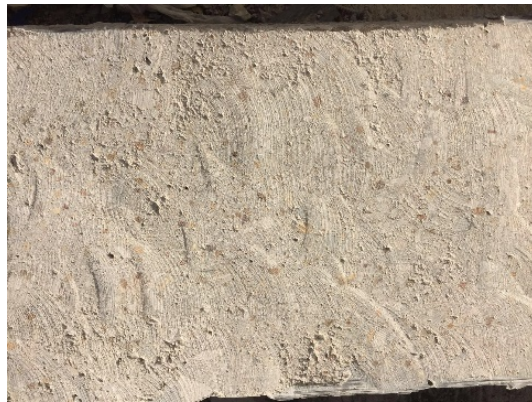
Figure 3-5a: Concrete surface roughness (CSP) 2 using hand grinding
