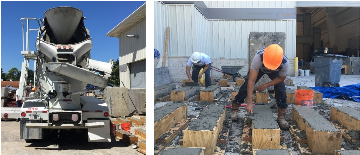
Figure 3-3: Casting of the concrete beams
