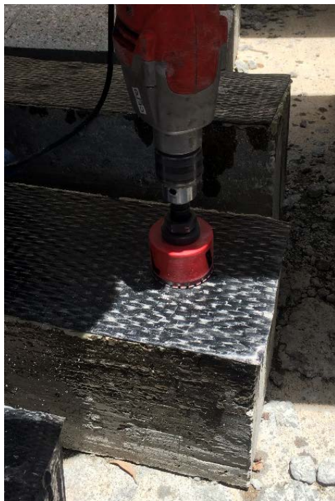
Figure 5- 4: Core drilling
