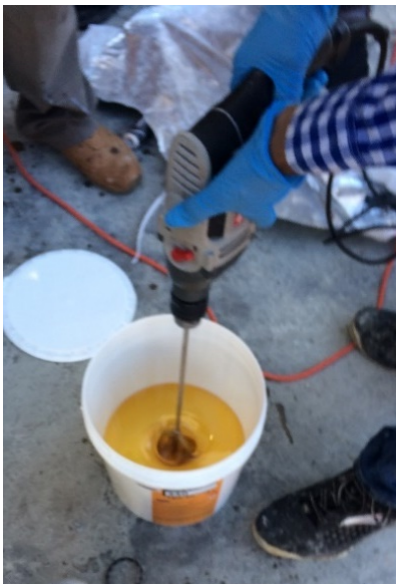
Figure 3-8: Mixing of the Epoxy
