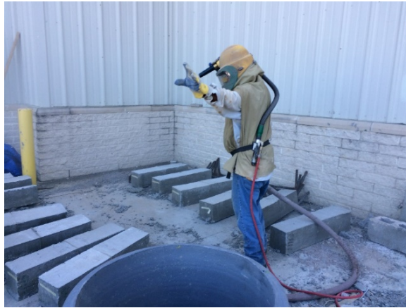
Figure 3-6a: Concrete surface preparation using sandblasting
