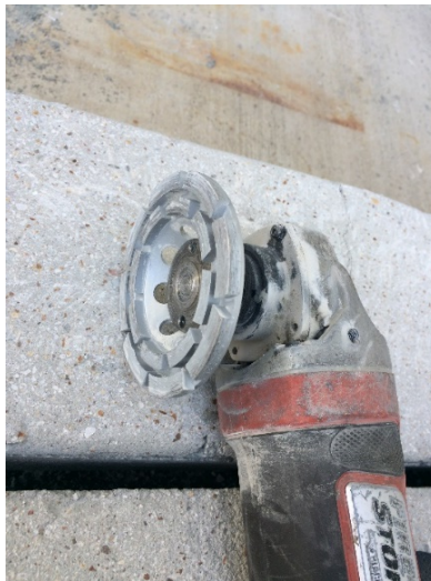
Figure 3-6b: Concrete surface preparation using hand grinding
