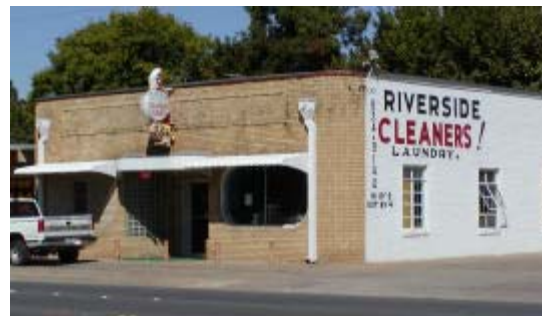
Early 20 th -century Riverside building
