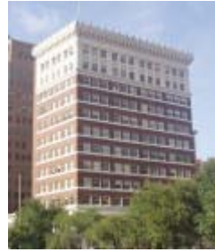
Burk Burnett Building
