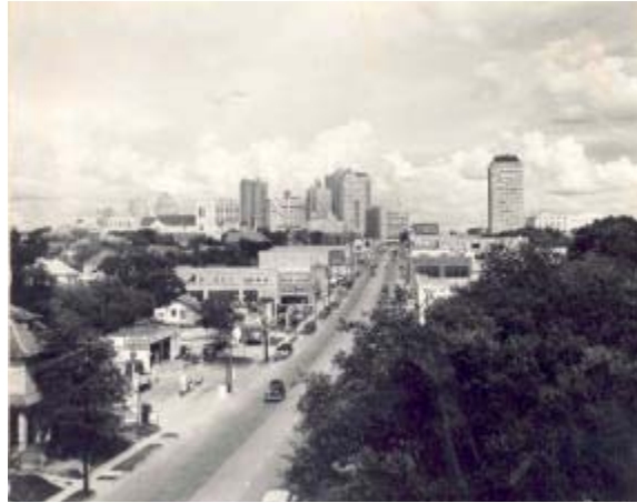
Historic commercial corridors are key areas for preservation and revitalization.
