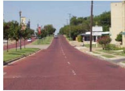
Camp Bowie Boulevard’s red brick paving
