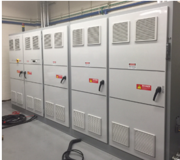
Figure 4.20: Photograph of UTA's 1200V/700A/500kW Chroma 17030 battery cycler.
