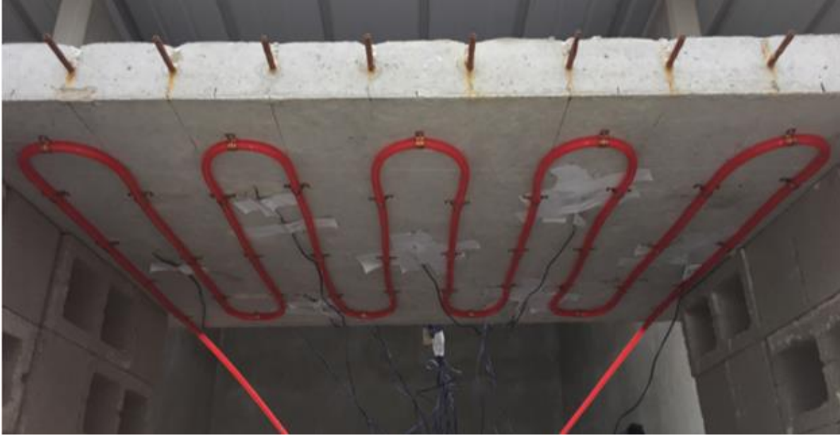
Figure 5- 2 Pipe Arrangement Prior to Framework Application
