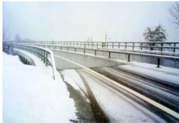
Figure 2- 19 SERSO system in operation (Eugster, 2007)
