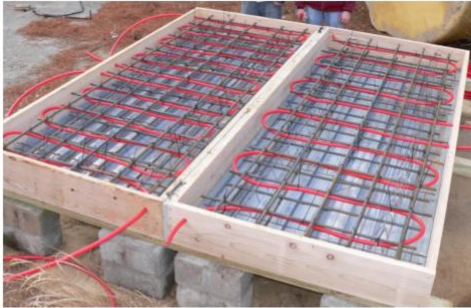
Figure 2- 7 Experimental Bridge Deck during Construction Process (Bowers, 2016)
