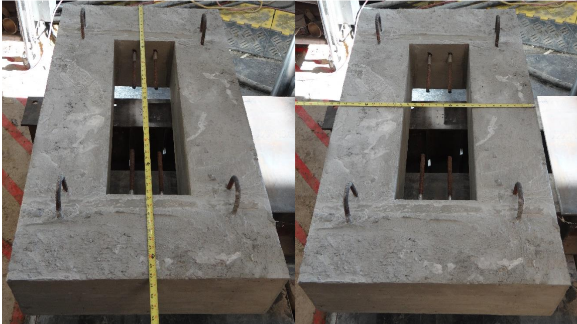
Figure 3- 20 Outer hollow slab showing embedded rebar location.
