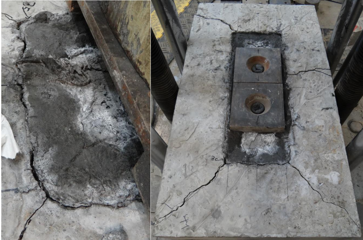
Figure 4- 26 Interface crack caused due to vertical slip and cracks observed on the outer support slab.
