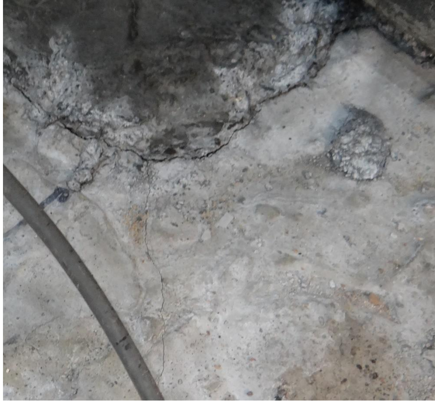
Figure 4- 24 Interface cracks observed in the UHP-FRC punch test specimen after peak.
