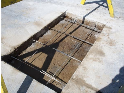
Figure 3- 11 Conventional concrete repair.
