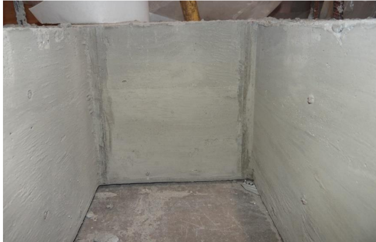
Figure 3- 18 Concrete surface roughness (cast in contact with wood formwork).
