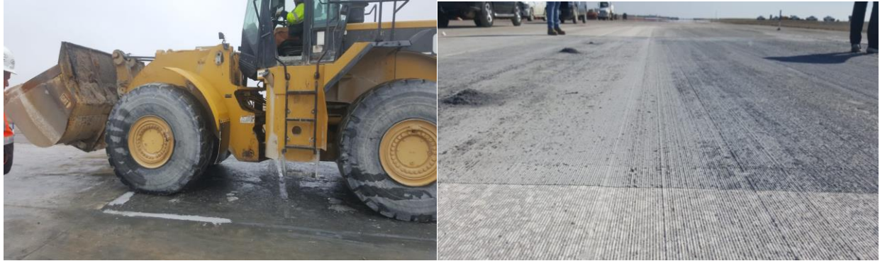
Figure 5- 13 Load testing of the UHP-FRC pavement repair site
