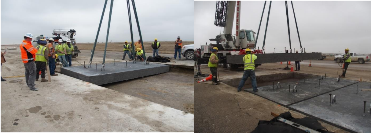
Figure 5- 10 Placement of the pre-cast UHP-FRC in the repair site
