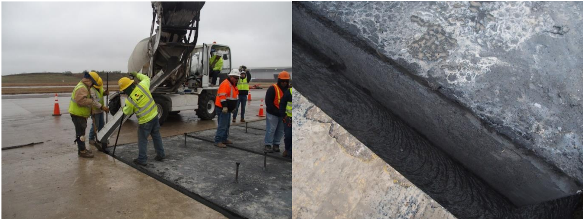
Figure 5- 11 Pouring of UHP-FRC cast-in-place joint
