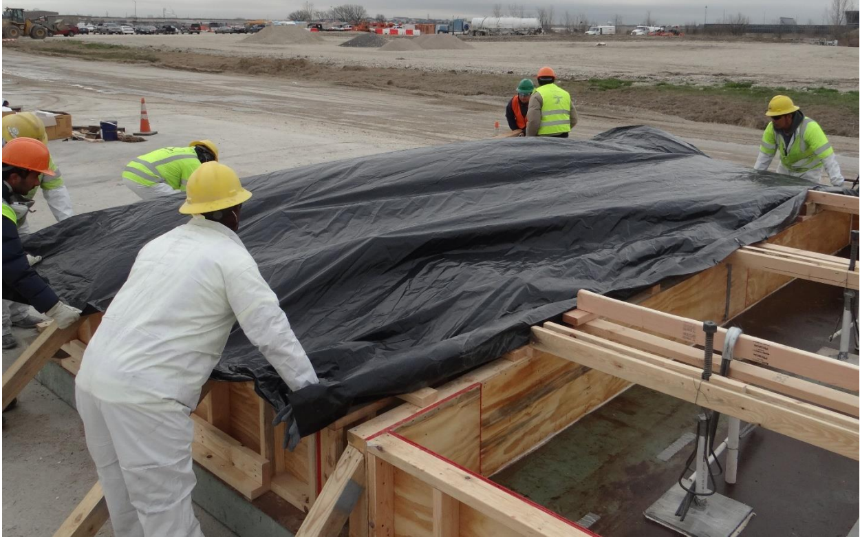
Figure 5- 8 Covering up of the UHP-FRC panel for curing
