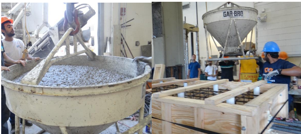
Figure 8- 25 Concrete pouring of the support block
