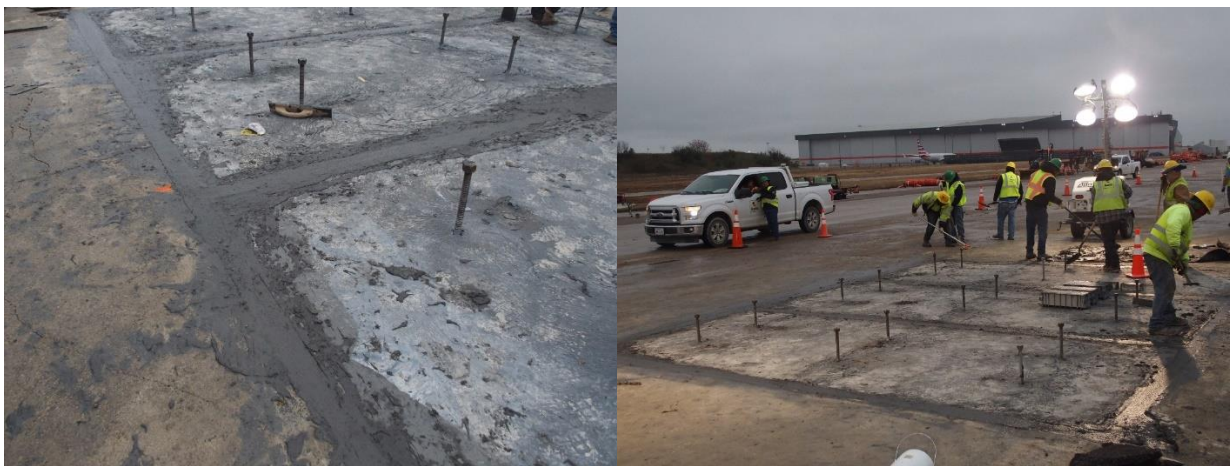
Figure 5- 12 The pavement after pouring of cast-in-place UHP-FRC joint
