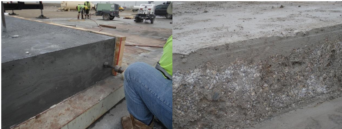
Figure 5- 9 Roughening of the UHP-FRC precast panels
