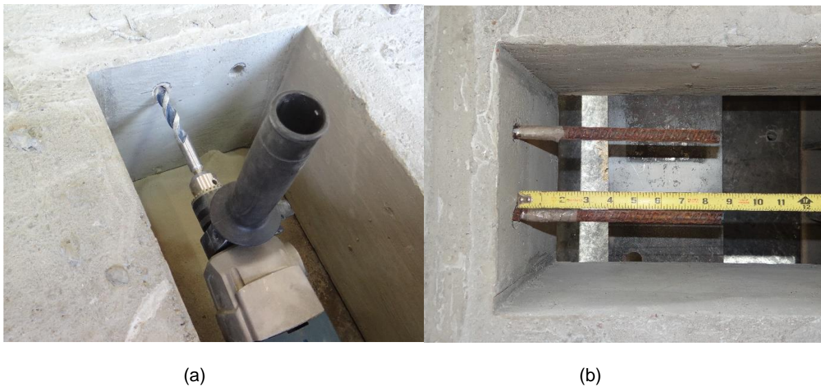
Figure 3- 19 (a) Drilling in the outer hollow slab for rebar placement and (b) rebar length inside the newly repaired concrete.
