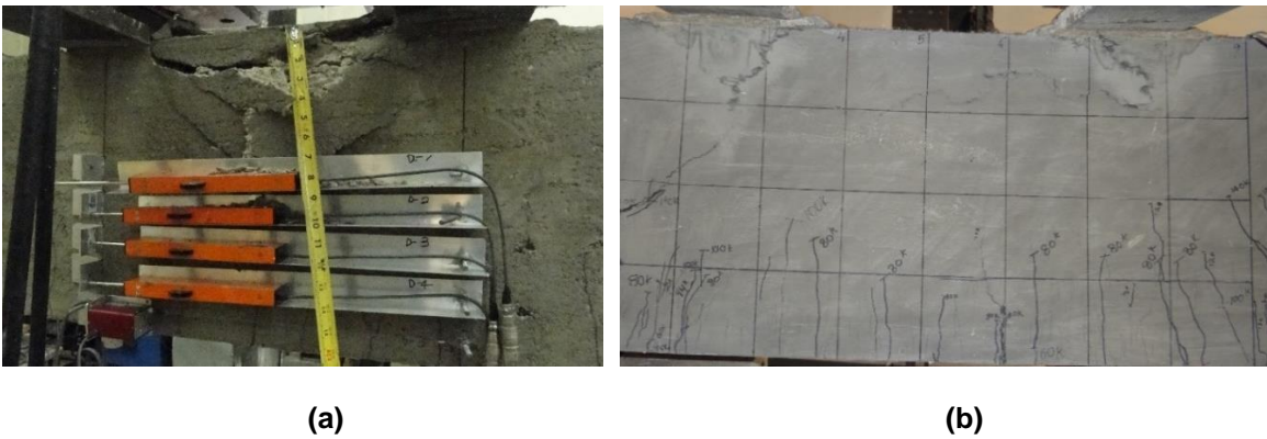
Figure 7- 20 Damage at end of testing: (a) RC beam; (b) UHP-FRC (with BFRP bars) beam without shear reinforcement
