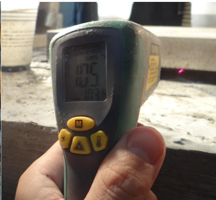
Figure 3- 29 The cast-in-place UHP-FRC repair joint heated to an average temperature of 100 °F using a combination of heaters.
