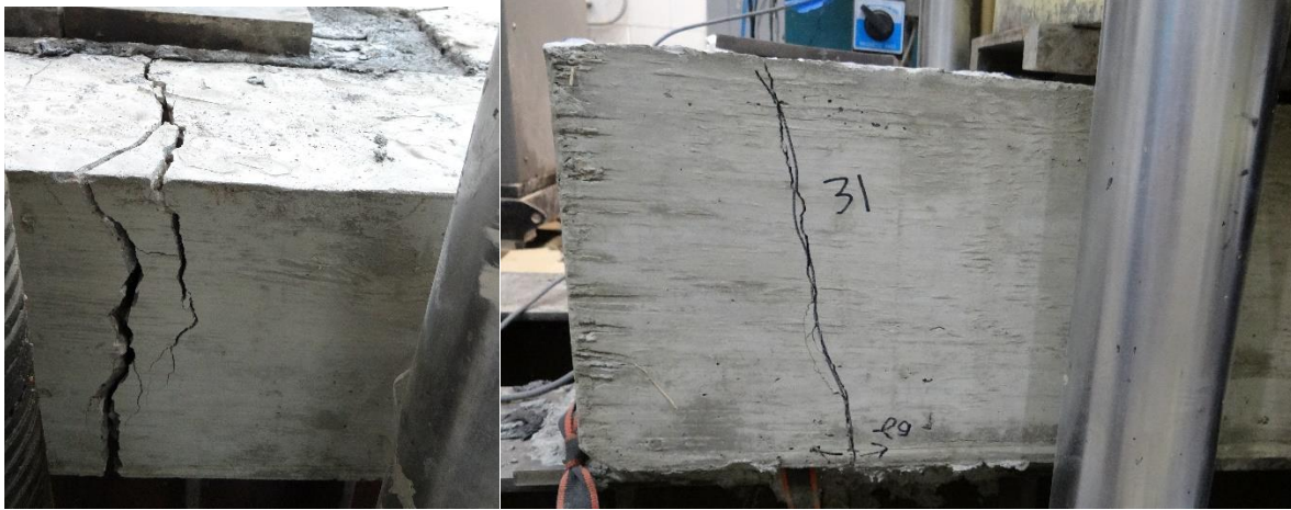
Figure 4- 28 Cracks at the mid-span and the edge of the support outer slab.
