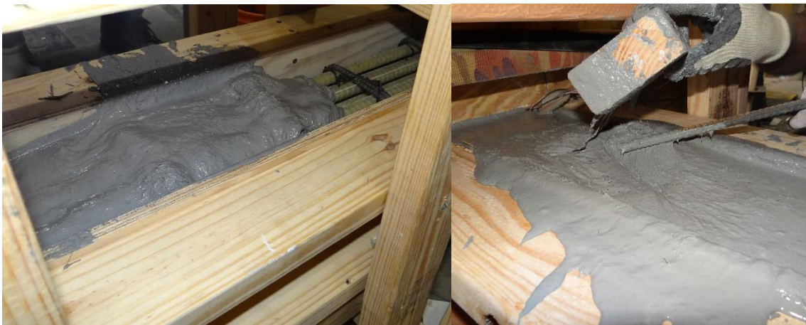
Figure 8- 29 UHP-FRC pouring for the specimens
