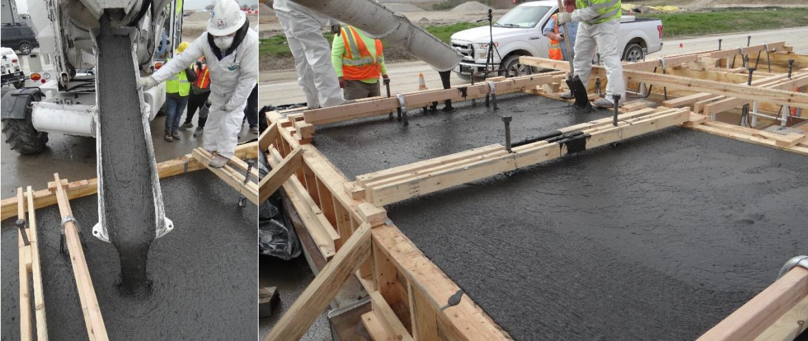
Figure 5- 6 Pouring UHP-FRC for the precast UHP-FRC panel
