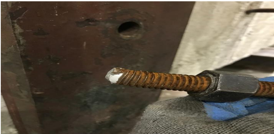
Figure 22: Anchor bolt after steel failure
