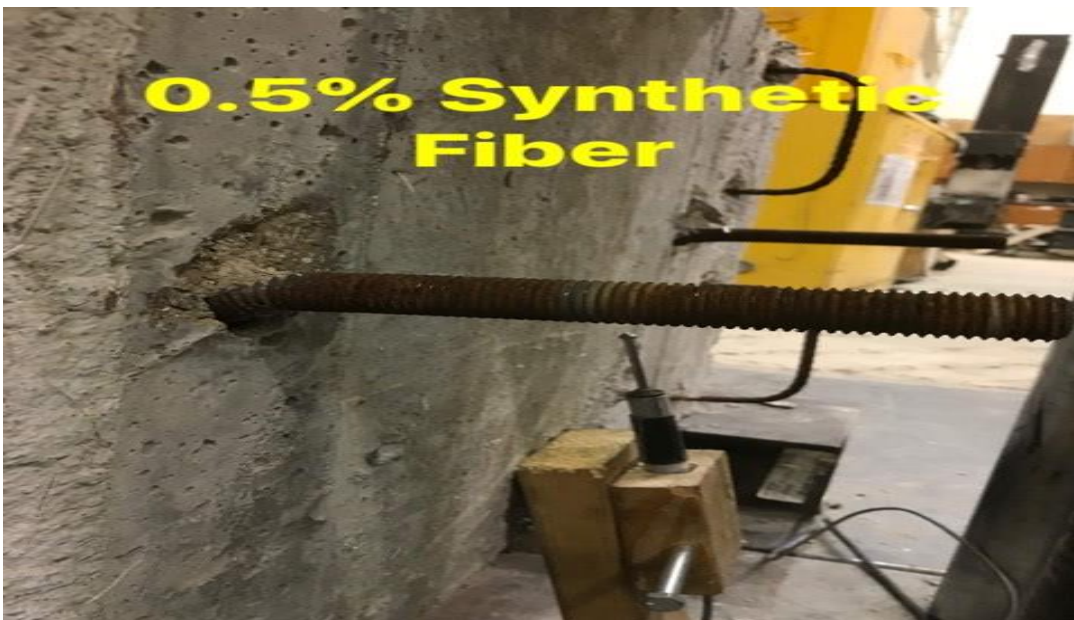
Figure 34: Steel failure preceded by concrete spall for 0.5% synthetic fiber
