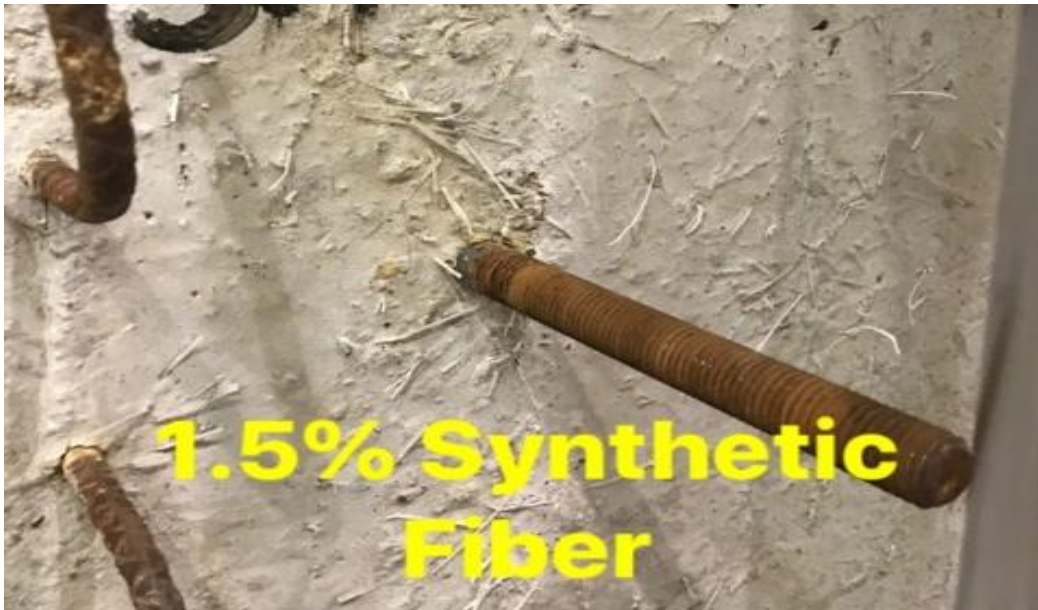
Figure 37: Steel failure preceded by concrete spall for 1.5% synthetic fiber
