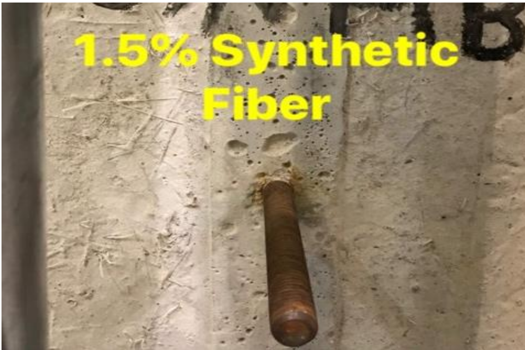
Figure 38: Steel failure preceded by concrete spall for 1.5% synthetic fiber
