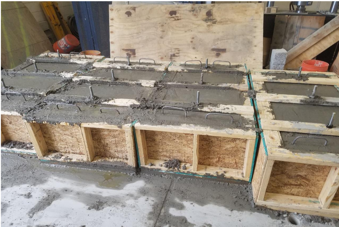
Figure 10: Large concrete beams after pour
