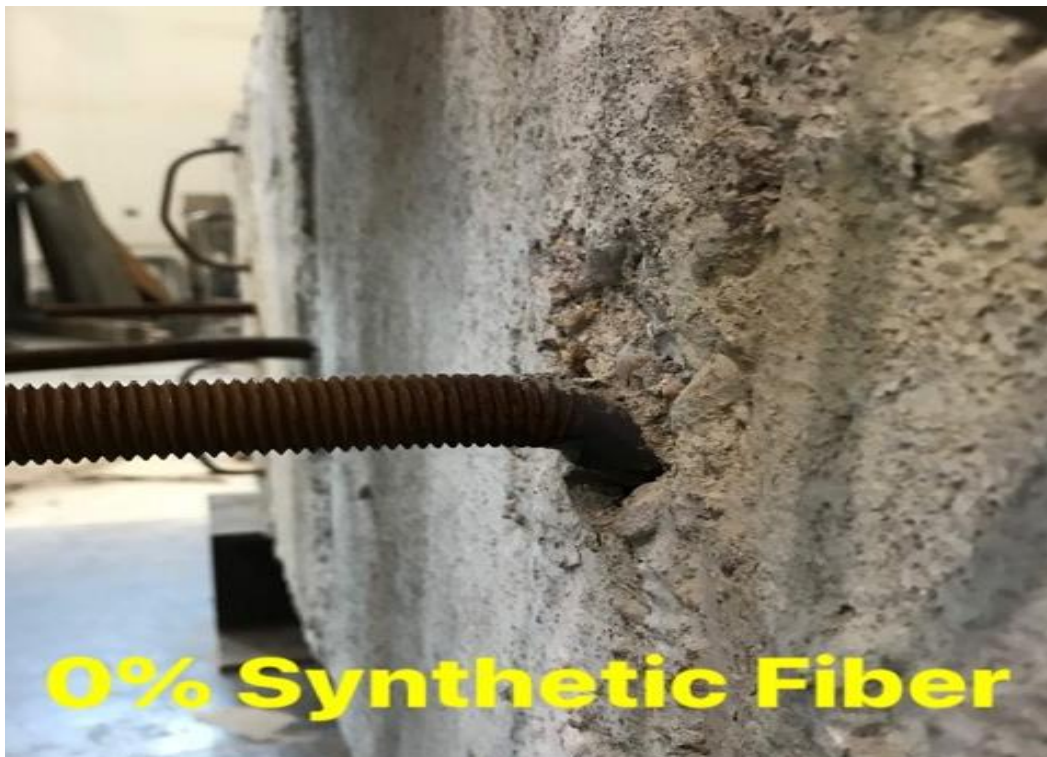
Figure 32: Steel failure preceded by concrete spall for 0% synthetic fiber
