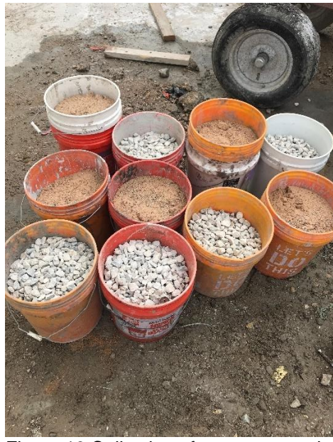
Figure 10 Collection of aggregates prior to mixing concrete
