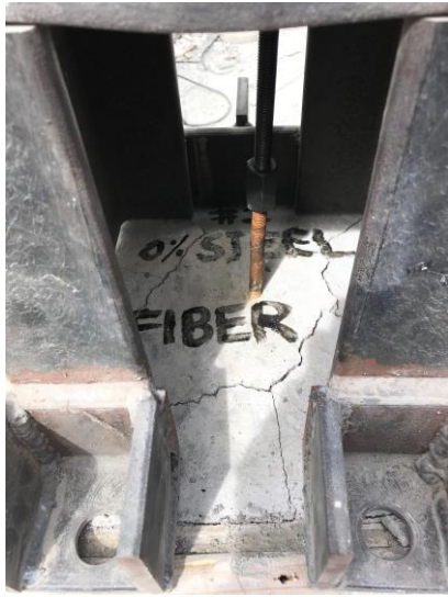
Figure 24 0.0% steel fiber reinforced concrete beam with embedded anchor bolt
