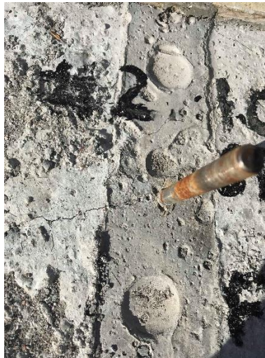
Figure 29: 1% steel fiber reinforced concrete beam with embedded anchor bolt after test #2 anchor
