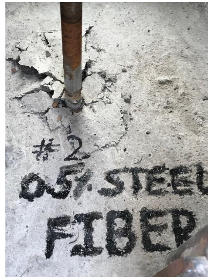
Figure 27 0.5% steel fiber reinforced concrete beam with embedded anchor bolt.
