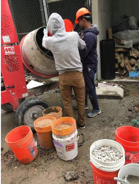
Figure 8 Pouring aggregates into the concrete mixer.
