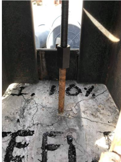
Figure 28: 1% steel fiber reinforced concrete beam with embedded anchor bolt after test #1 anchor
