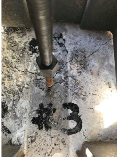
Figure 30: 1% steel fiber reinforced concrete beam with embedded anchor bolt after test #3 anchor
