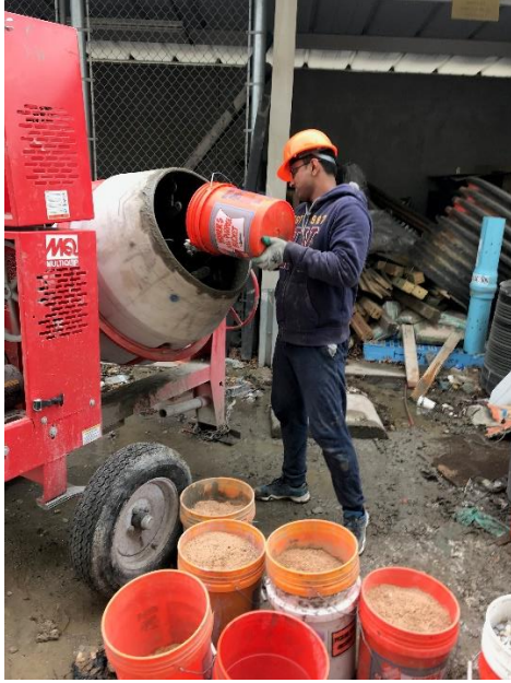
Figure 7 Pouring aggregates into the concrete mixer.
