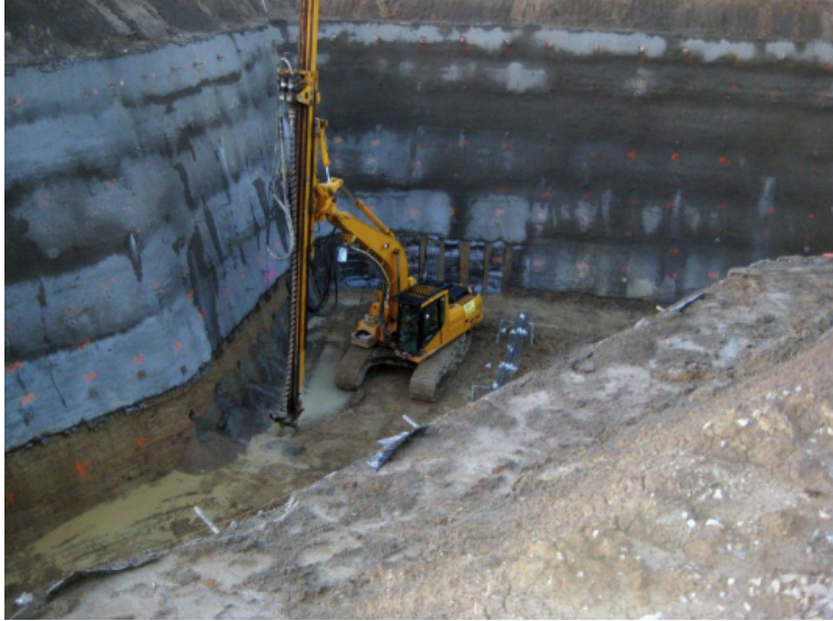
Figure 2- 7 Soil Nail wall construction (Source: HaywardBaker.com)
